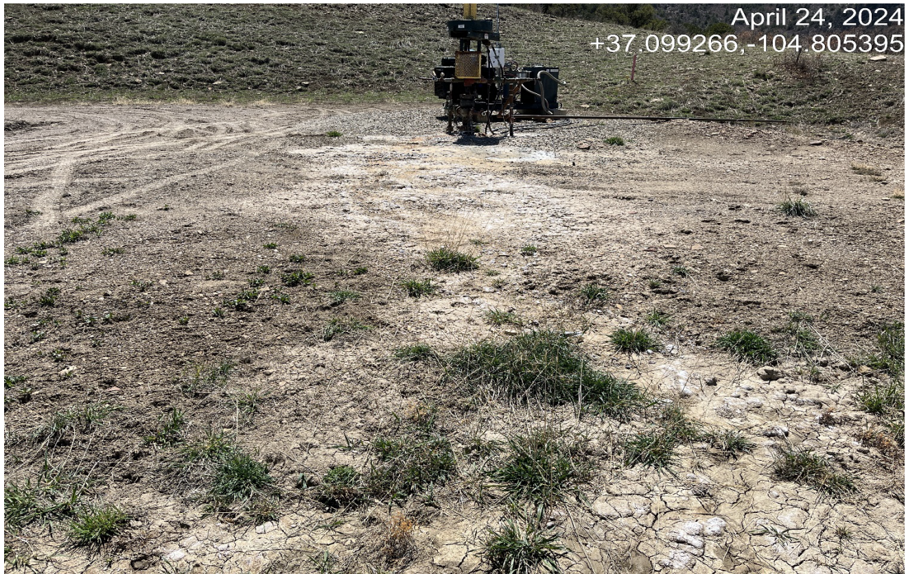
Photo 2. It appears there was a produced water leak at the wellhead that that flowed north toward the fill slope.
