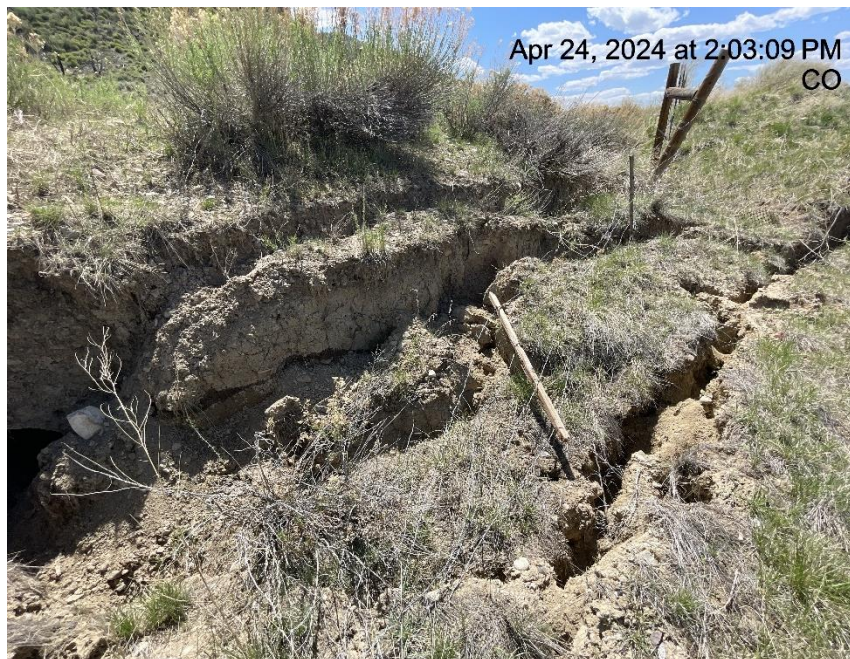
Photo # 4895 Slope destabilized & sloughing
