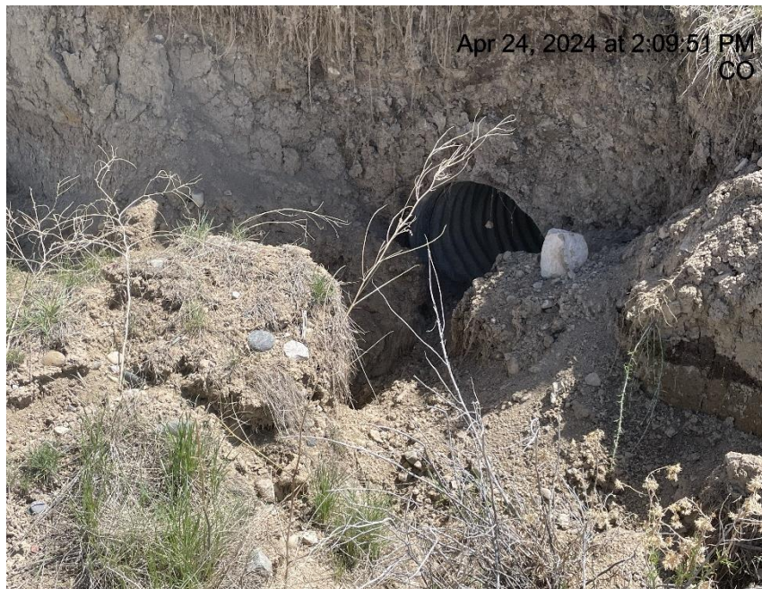
Photo # 4889 Culvert damaged/BMP needs maintenance
