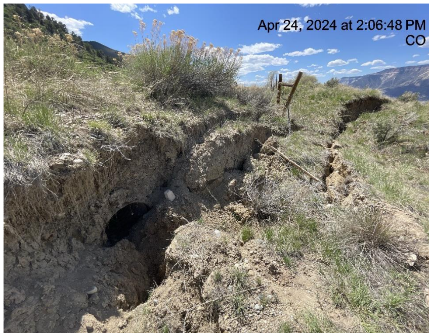
Photo # 4887 Culvert damaged/BMP needs maintenance
