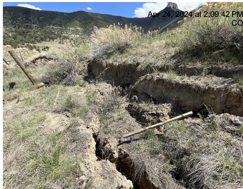
Photo # 4896 Slope destabilized & sloughing
