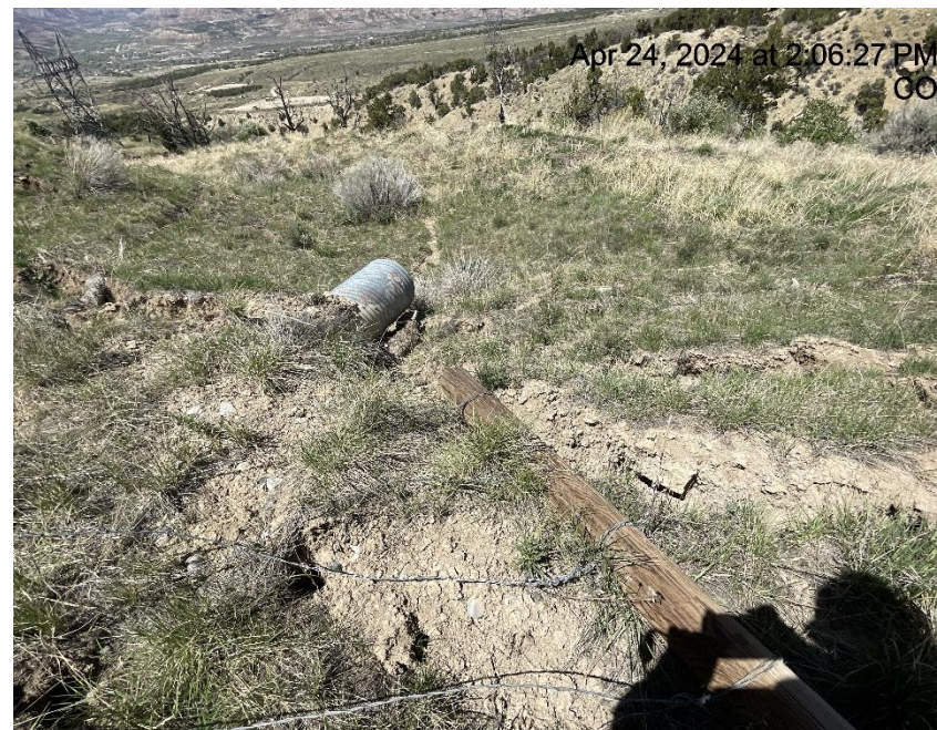
Photo # 4888 Culvert damaged/BMP needs maintenance
