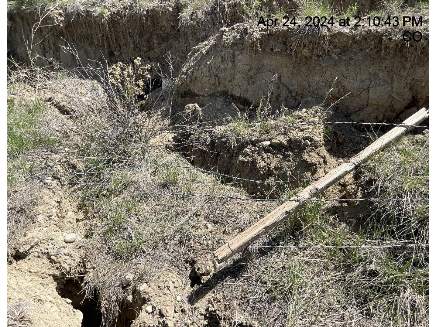
Photo # 4880 Barbed wire fence needs maintenance, barbed wire laying on ground/wildlife hazard
