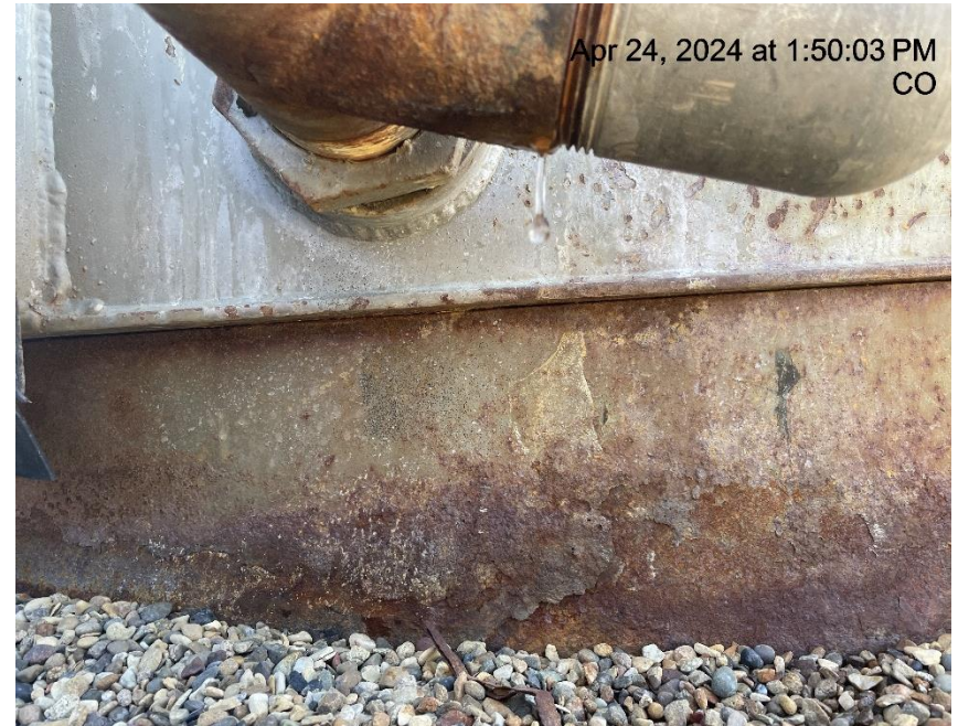
Photo # 4884 Mechanical condition - fluid leaking from tank valve
