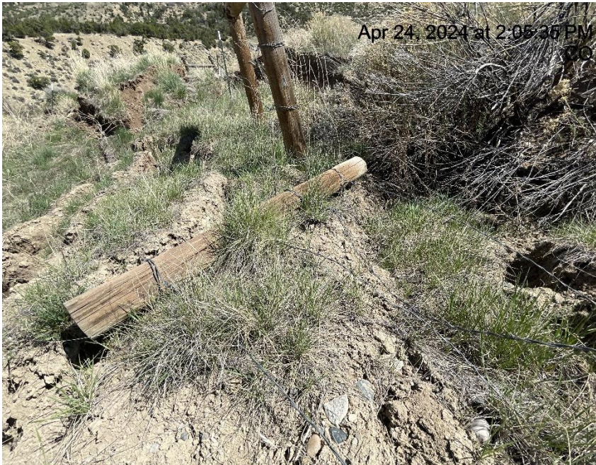
Photo # 4881 Barbed wire fence needs maintenance, barbed wire laying on ground/wildlife hazard
