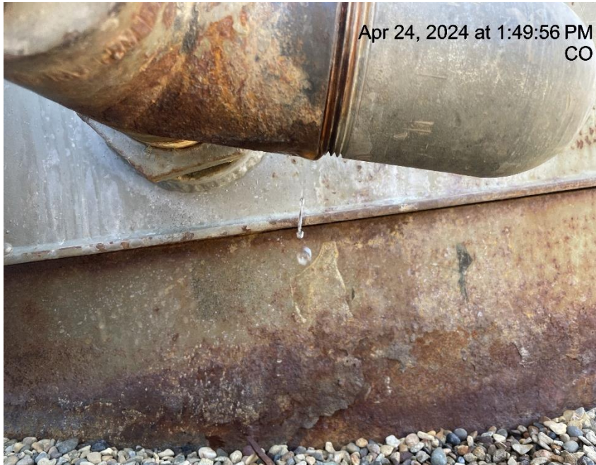
Photo # 4883 Mechanical condition - fluid leaking from tank valve
