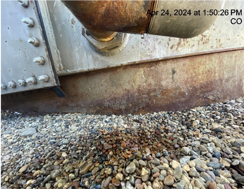
Photo # 4885 Mechanical condition - fluid leaking from tank valve
