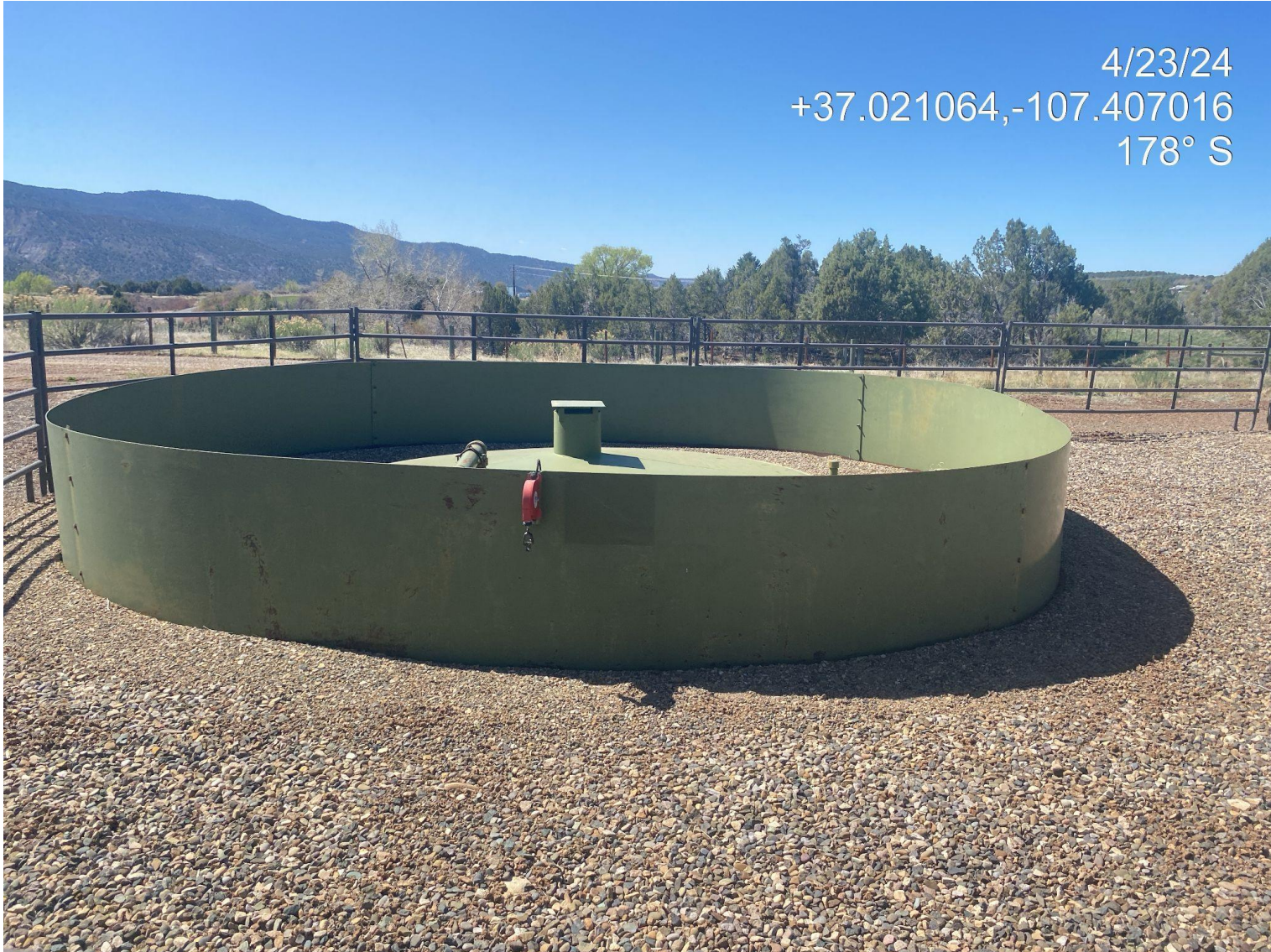
Photo 2. No sign/placard observed for produced water tank.
