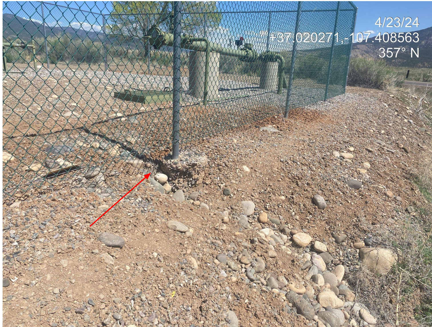
Photo 4. View of rill erosion forming and under cutting fence line on location.
