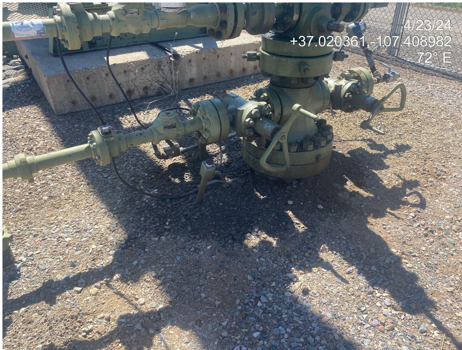
Photo 2. Impacted surface material observed at well head.
