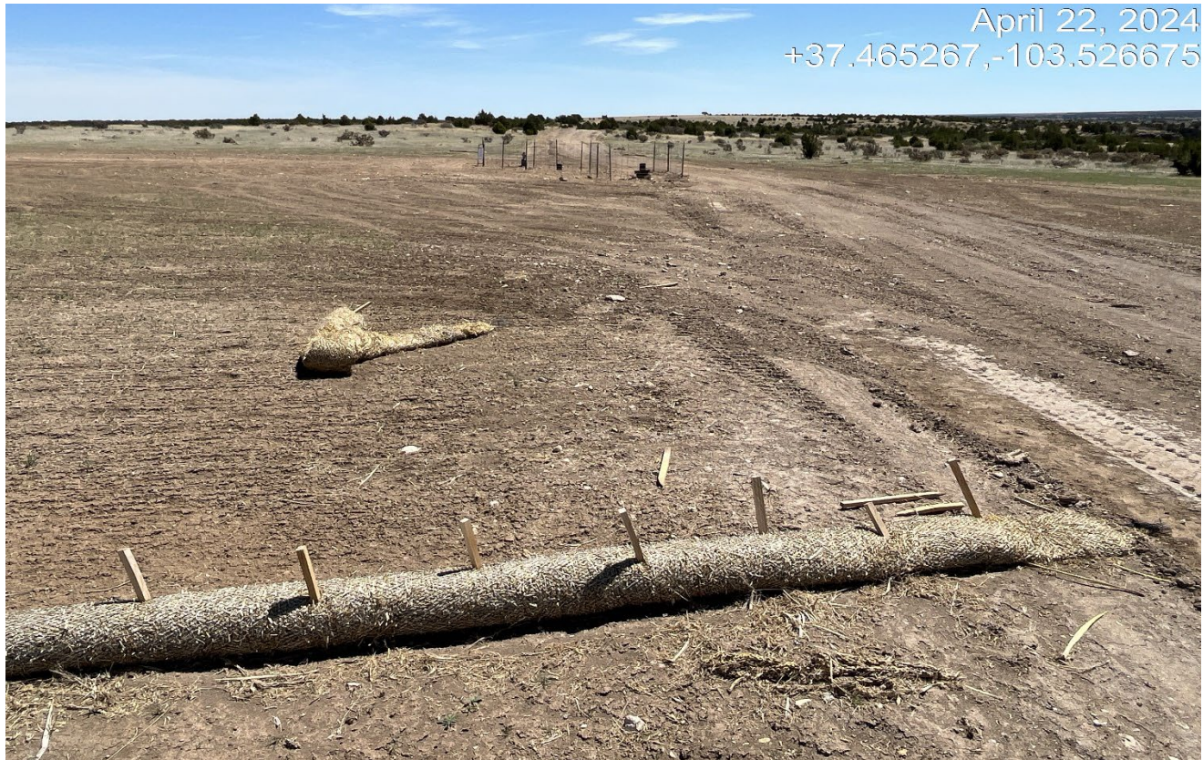
Photo 8. Facing east at the location. The stormwater wattles are displaced and have been run over by vehicles .
