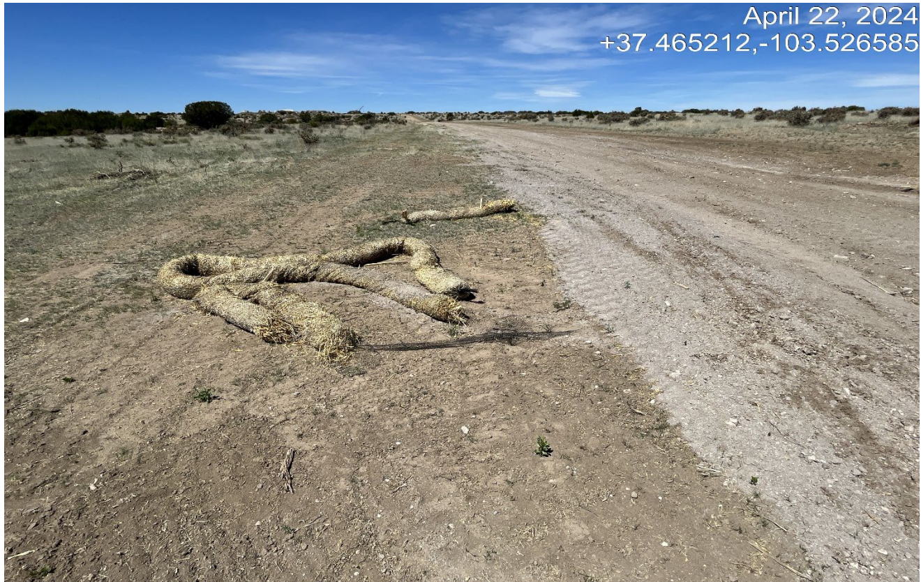
Photo 6. West side of the location. The are broken up straw wattles that need to be removed.
