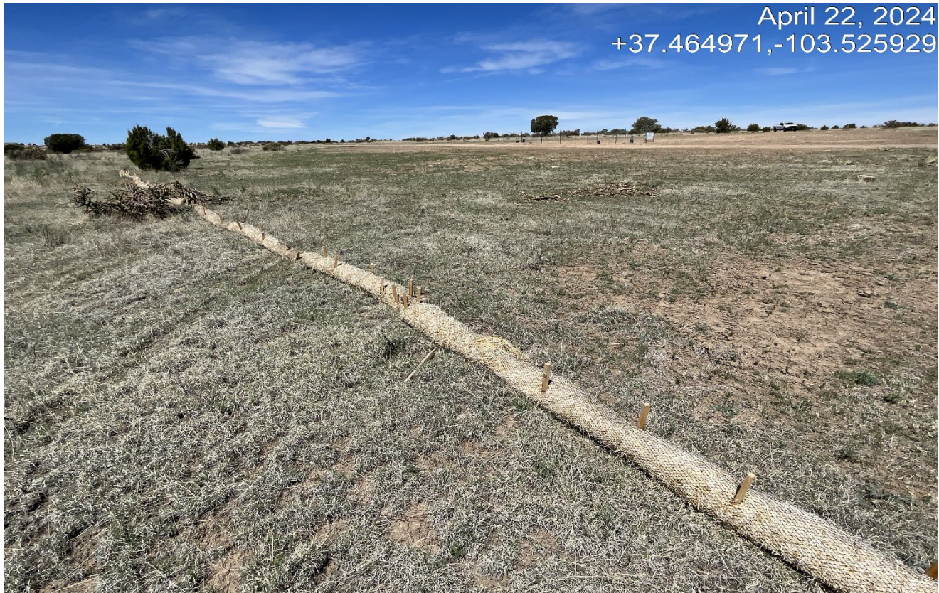
Photo 5. Facing northwest at the location. These perimeter wattles are installed far away from the disturbance area and should be reinstalled for better erosion control.
