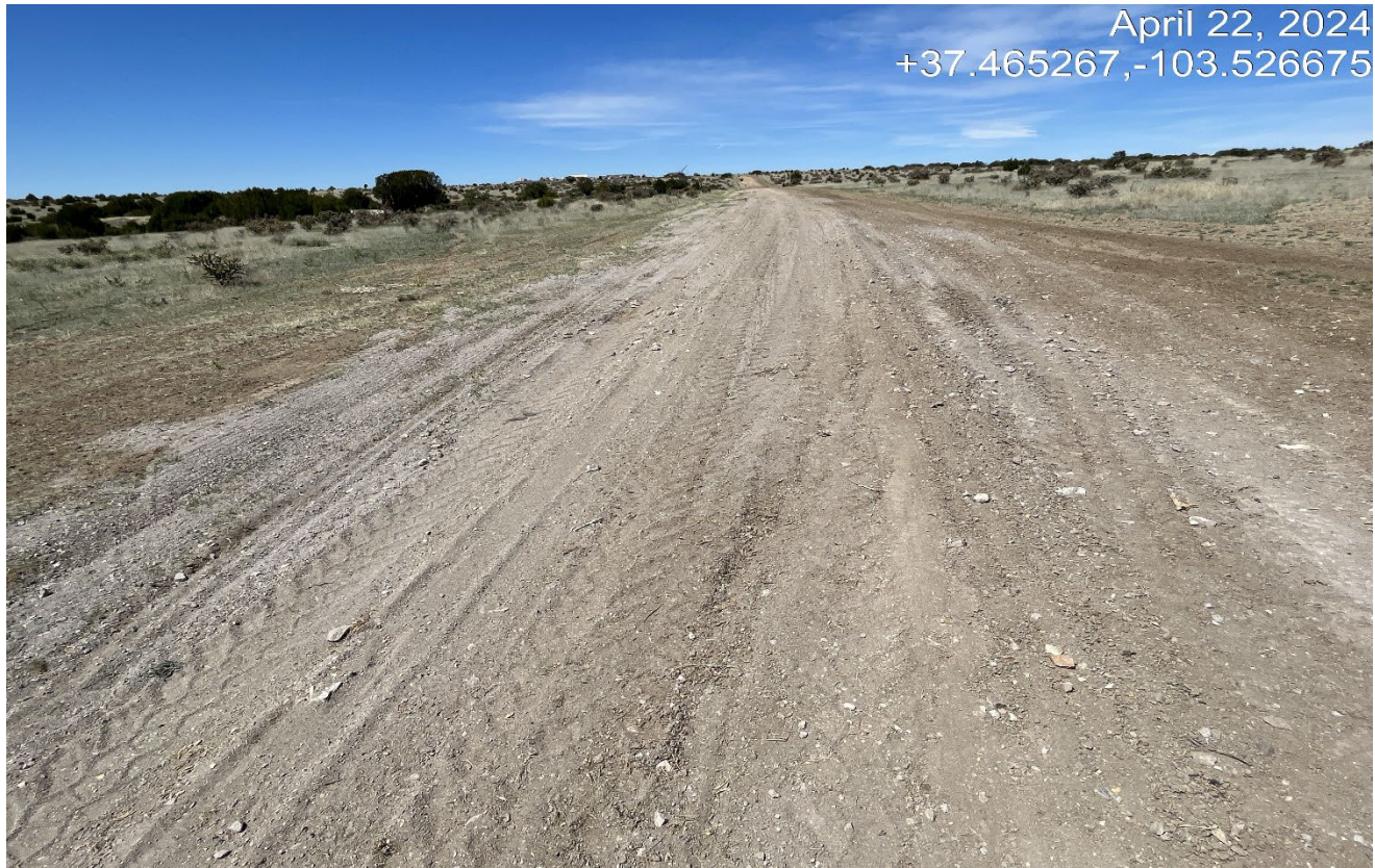
Photo 7. Facing west toward the flowline disturbance. The topsoil was not salvaged along the flowline and grey material was brought to the surface. It is likely soil amendments or topsoil will be needed for reclamation.
