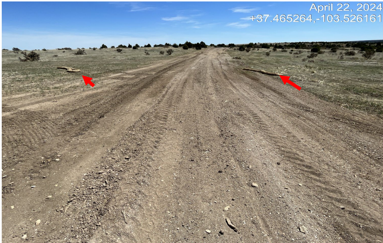
Photo 4. Facing east toward the flowline disturbance. The soils are not stabilized and are susceptible too erosion. There are displaced wattles shown at red arrows.
