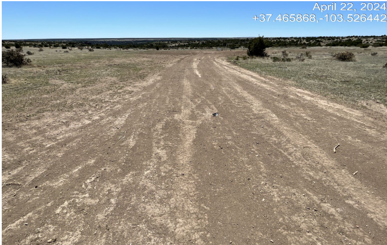
Photo 1. Facing south along the access road. Topsoil was not salvaged along the road and soils are very compacted.
