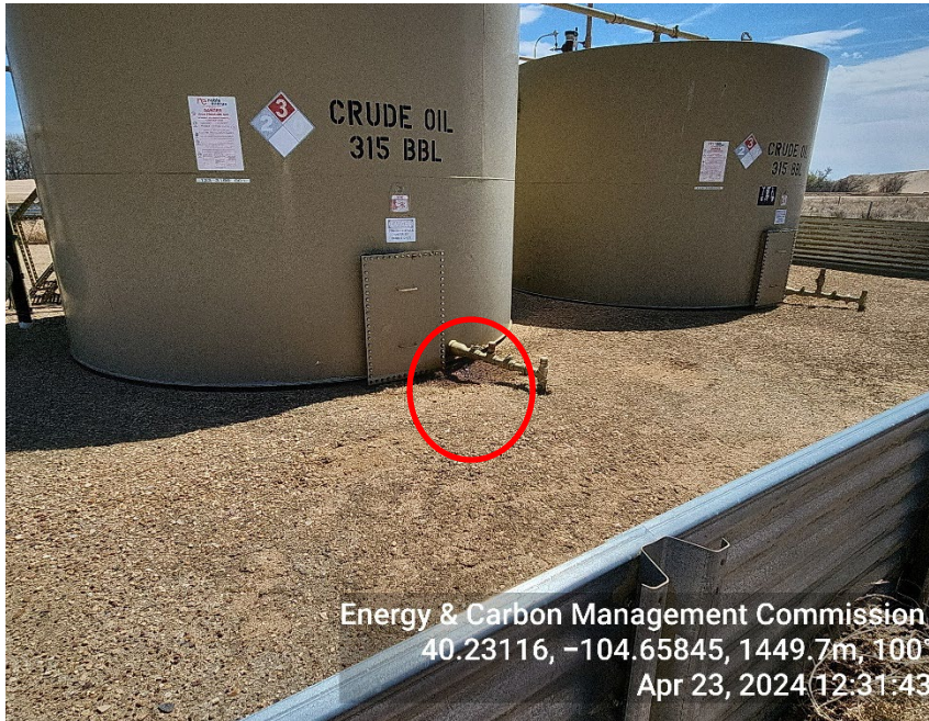
Photo 23: Leaking tank
