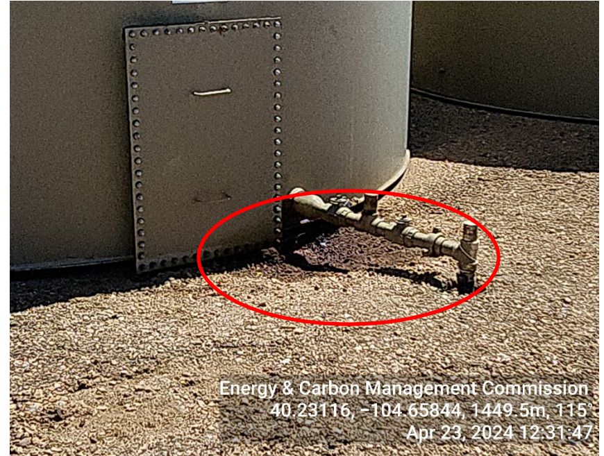
Photo 24: Leaking tank
