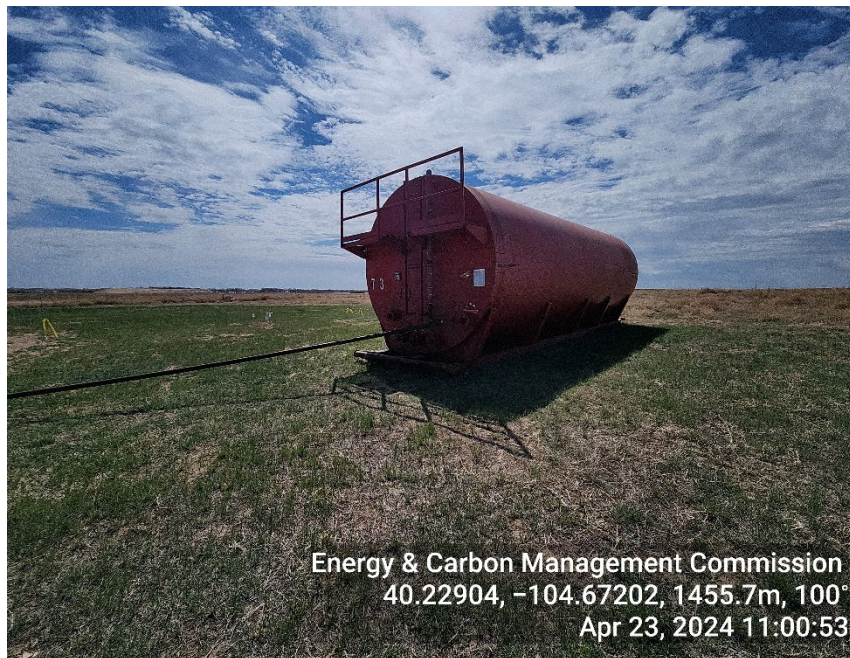
Photo 5: No grounding rod/berm
