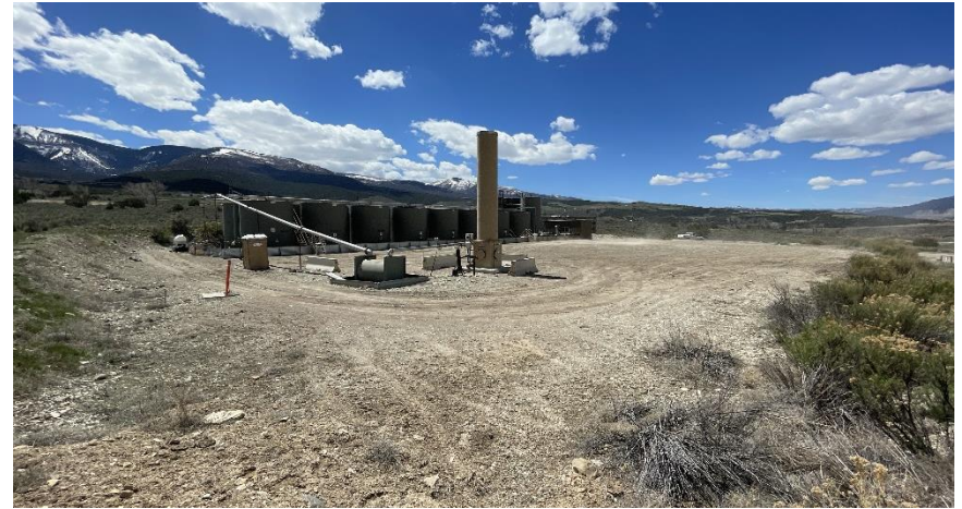
North East corner of location.
