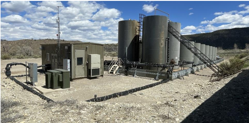
South West corner of location.
