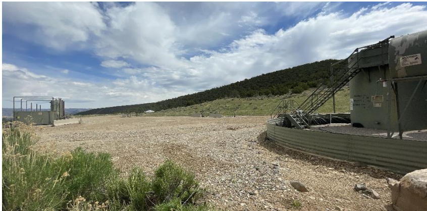
South West corner of location.
