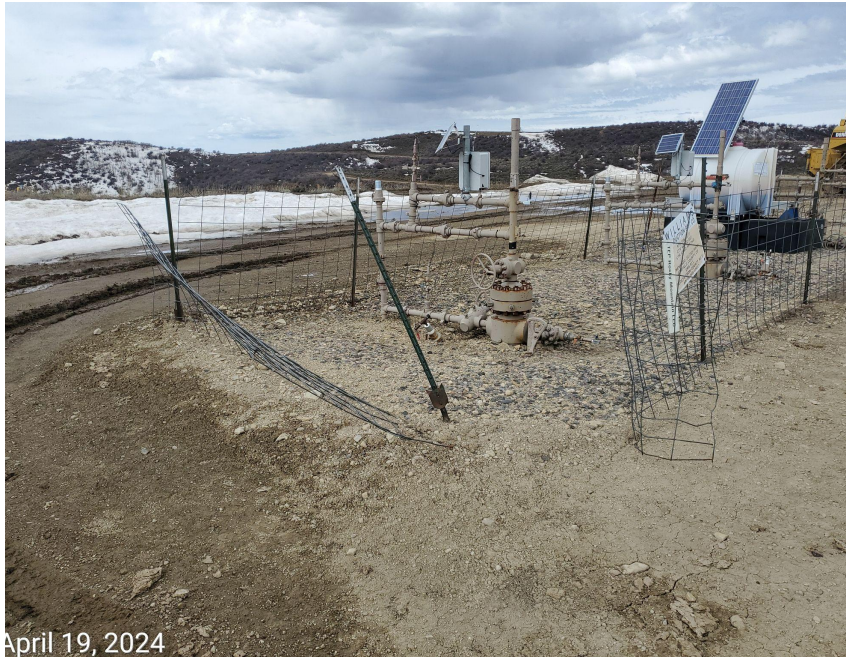
Photo 6: Fence in disrepair at wells, tank battery and separators.
