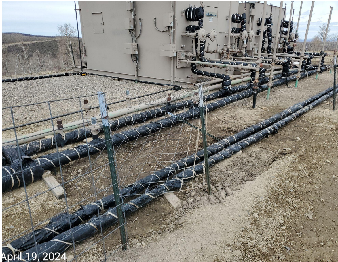
Photo 7: Fence in disrepair at wells, tank battery and separators.
