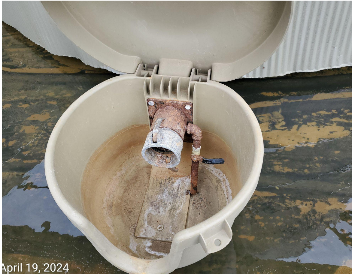
Photo 5: Photo example showing lines at tanks missing required cap/plug.
