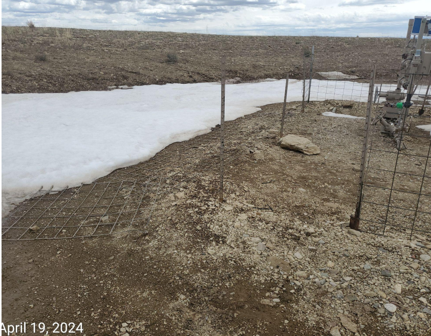
Photo 5: Photos examples showing fence at wells and separator equipment is in disrepair.
