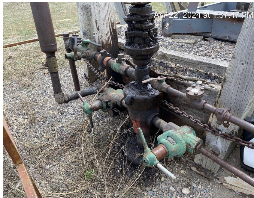
Stained soil on and around wellhead.
