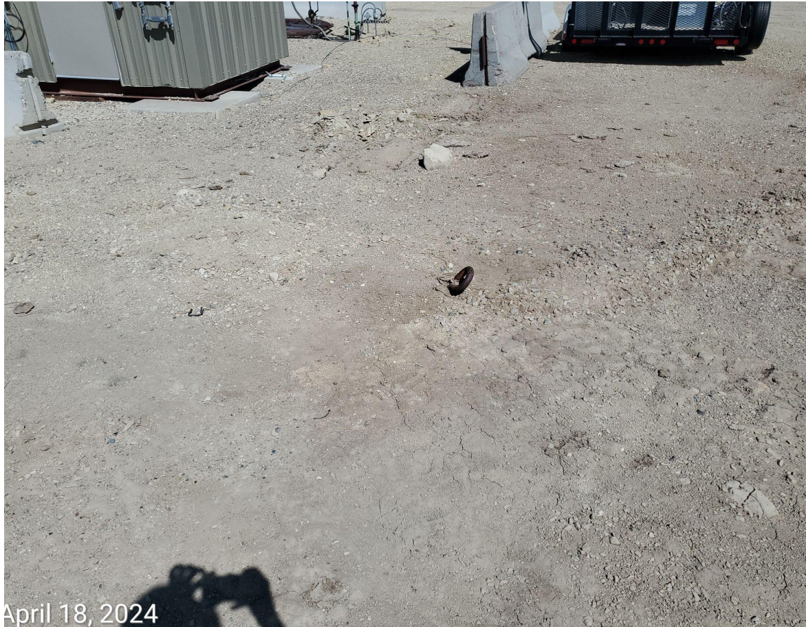
Photo 4: Photo example showing anchors on the Location observed missing required marking.
