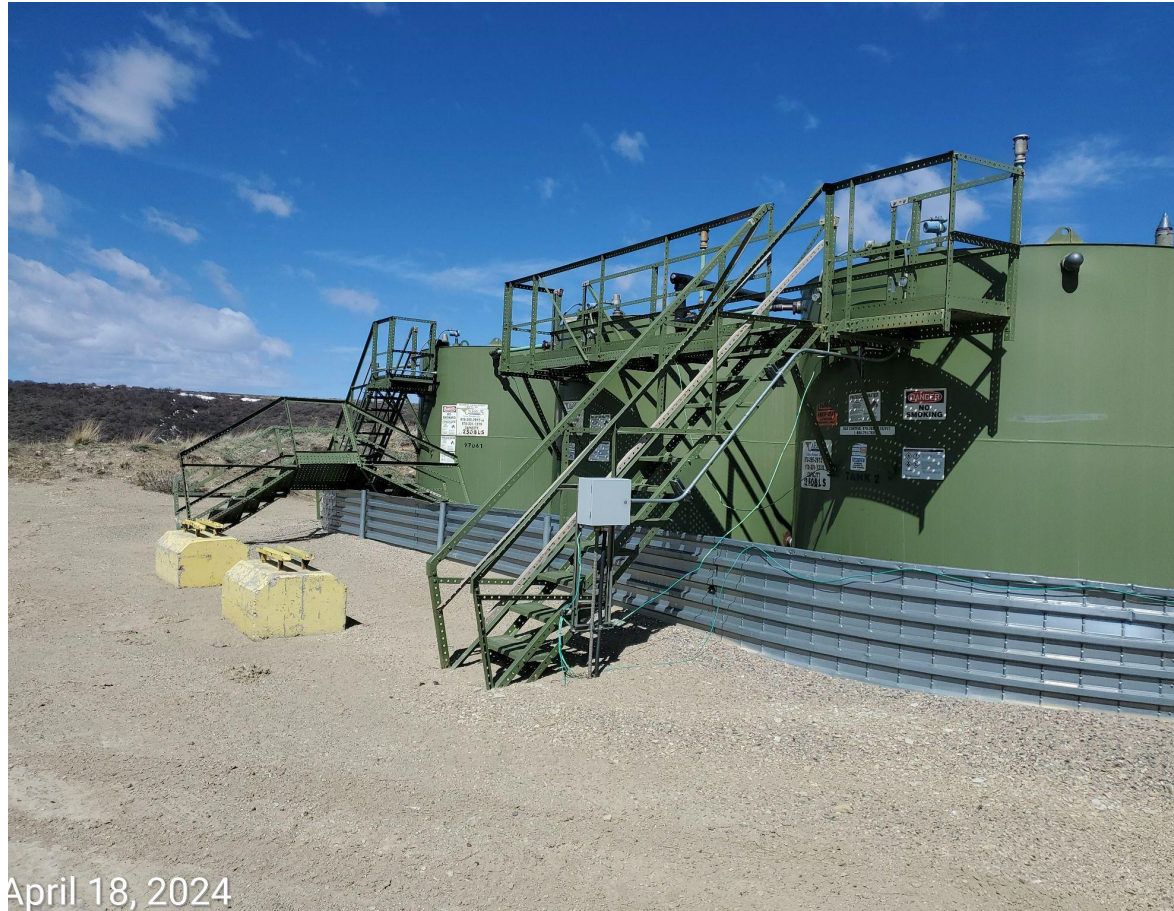
Photo 5: Tank battery facility missing signage per Rule 605.e.
