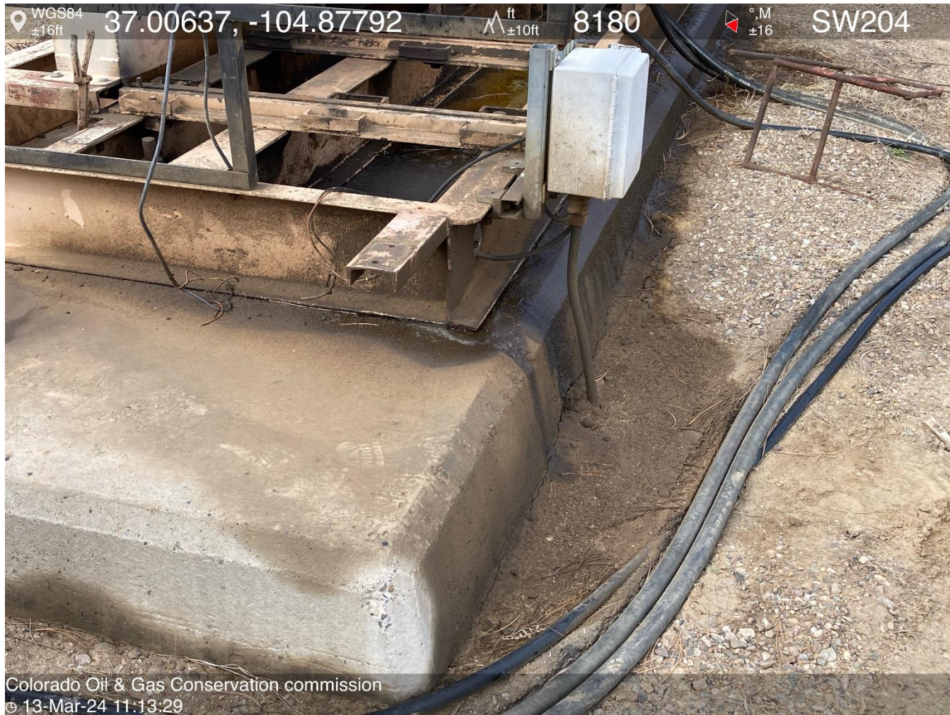
PHOTO 4: Impacted soil identified at various locations through out location. Conduct maintenance on equipment, cleanup stained material and review self inspection processes. COMPLY WITH RULE 1002,(2).D. CA DATE 5-22-24.
