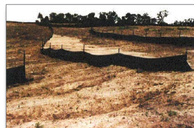
Figure 2. Create manageable sediment storage areas
