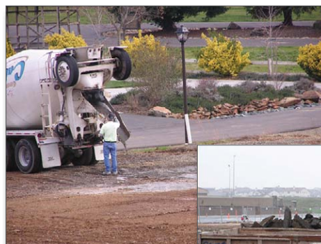
Figure 1. Chute washwater being dumped on the ground
