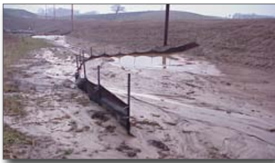
Figure 22. A silt fence full of sediment that needs maintenance
