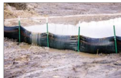
Figure 3. Water should not flow over the filter fabric during a normal rainfall
