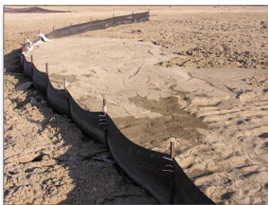
Figure 1. Silt fence retaining sediment
