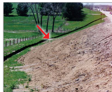
Figure 4. Avoid long runs of silt fence
