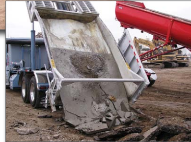
Figure 15. Delivering hardened Concrete to a recycler
