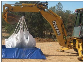
Figure 12. Extracting the concrete solids or gelled washwater
