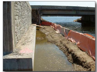
Figure 19. Silt fence for bridge abutment excavation
