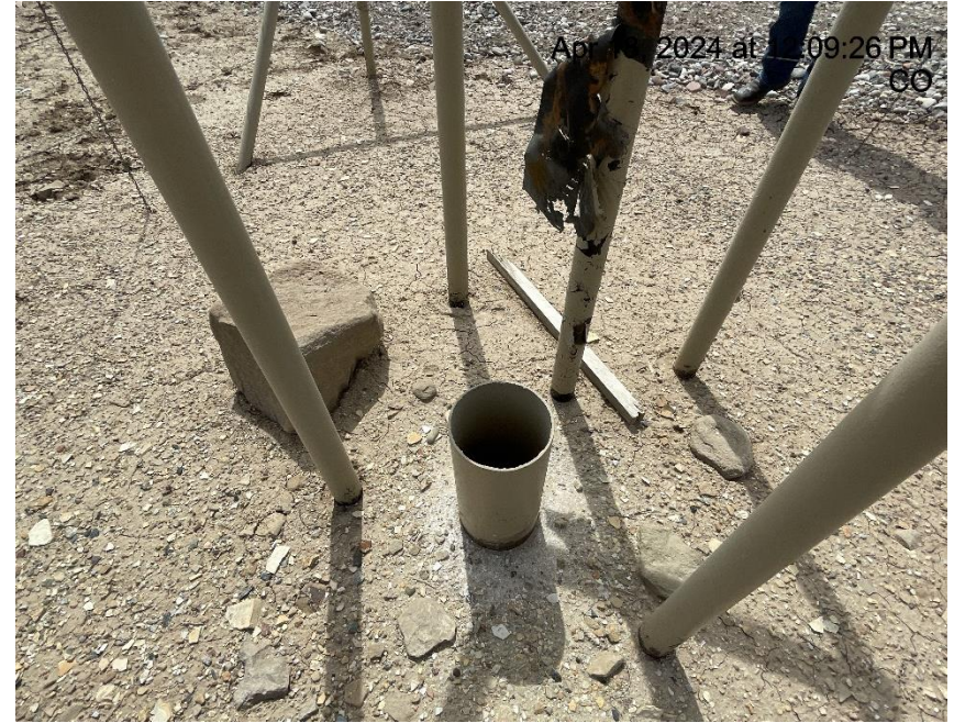
Photo # 4342 Open ended pipe/wildlife hazard
