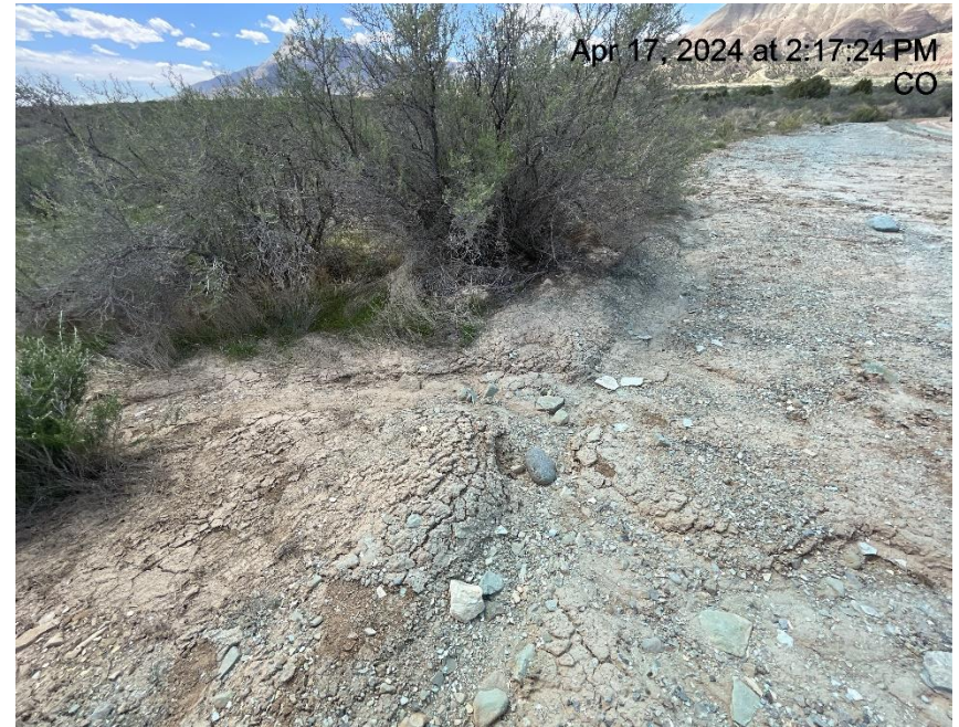
Photo # 4296 Berm needs maintenance/erosion & transport of sediment off location into a vegetated area (W/SW area of location)
