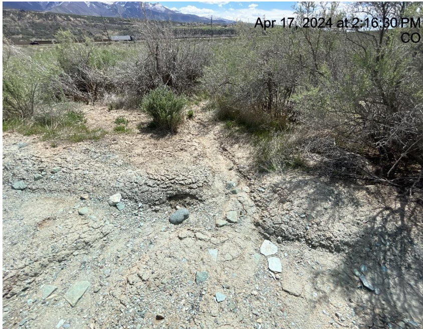
Photo # 4295 Berm needs maintenance/erosion & transport of sediment off location into a vegetated area (W/SW area of location)
