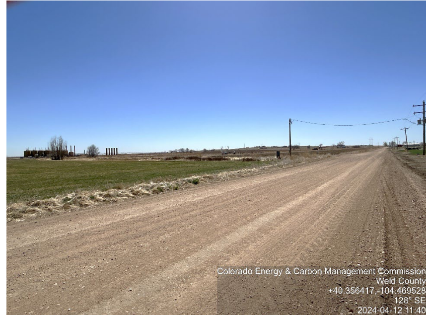
Photo #2 Siebring/5-63-32 South Pad Battery site Active Battery entrance
