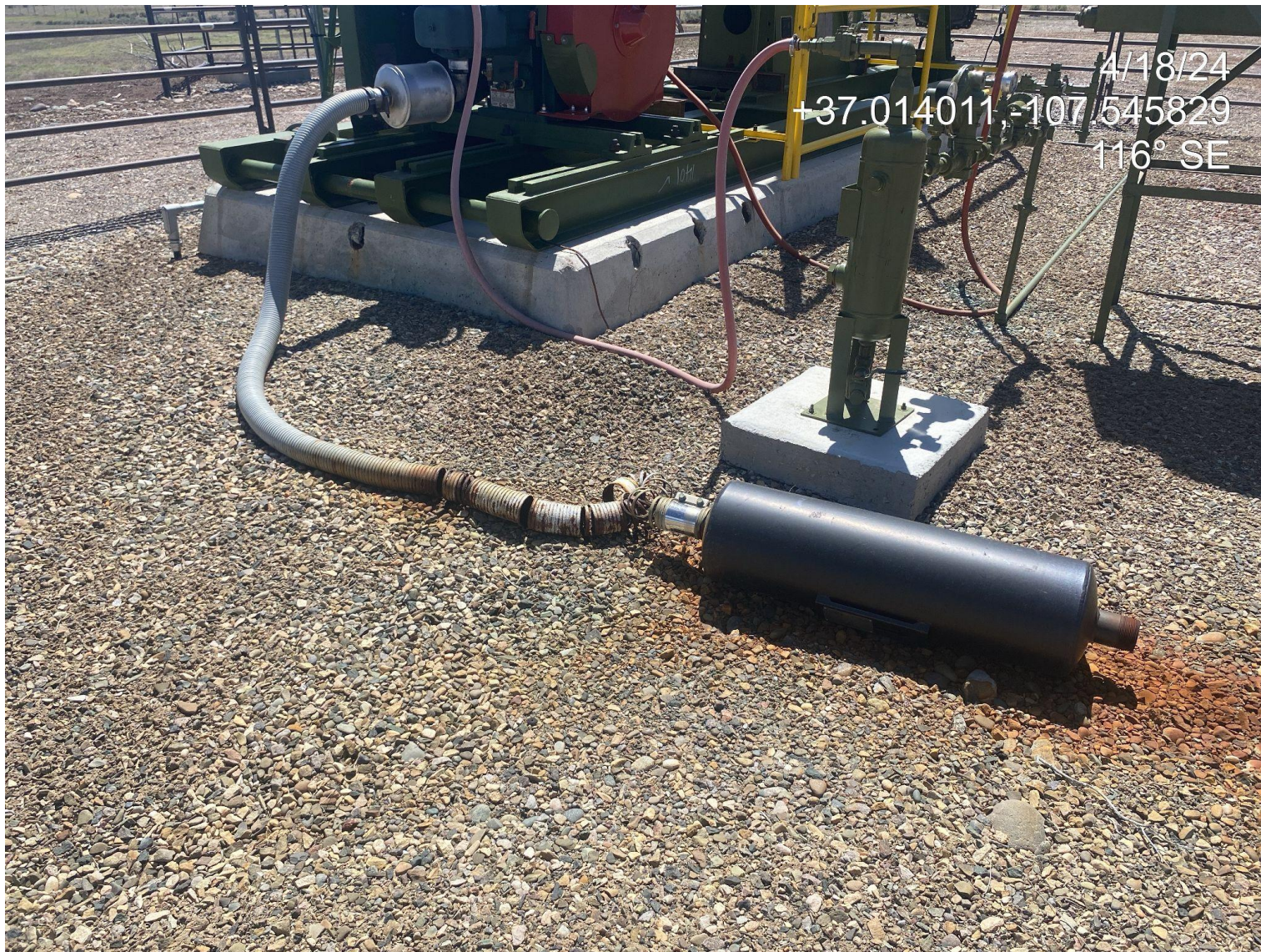
Photo 4. View of deteriorating muffler pipe impacting surface material.
