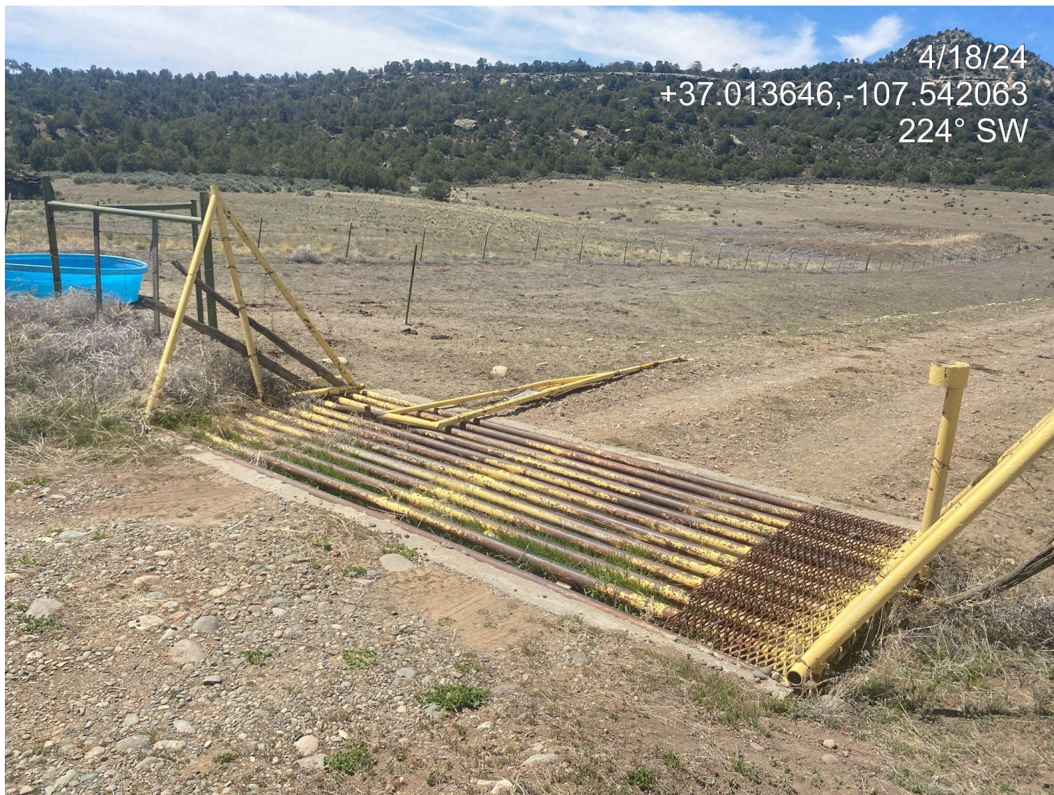
Photo 5. View of damaged access gate, maintenance is required.
