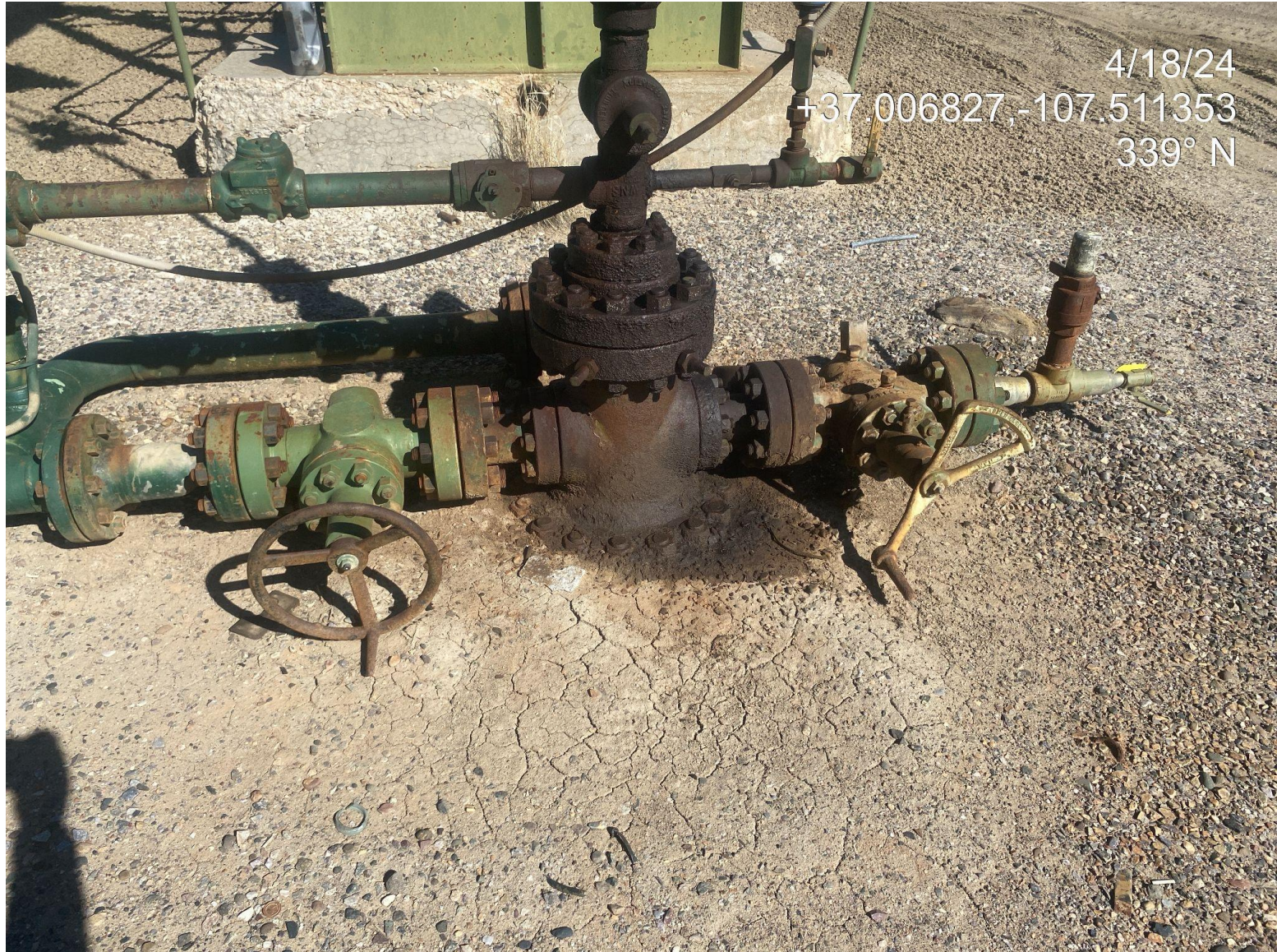
Photo 6. Impacted surface material observed at the well head.
