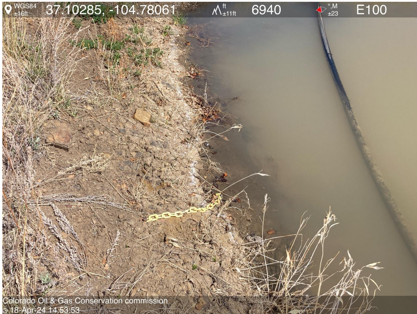
PHOTO 4: FLUID LEVEL IN PRODUCED WATER PIT IS ABOVE FREEBOARD (SPOKE WITH EVERGREEN PRODUCTION FOREMAN ED ROMERO). Lower fluid level so at least two feet of freeboard exists per Rule 909.c CA DATE 4/18/2024.
