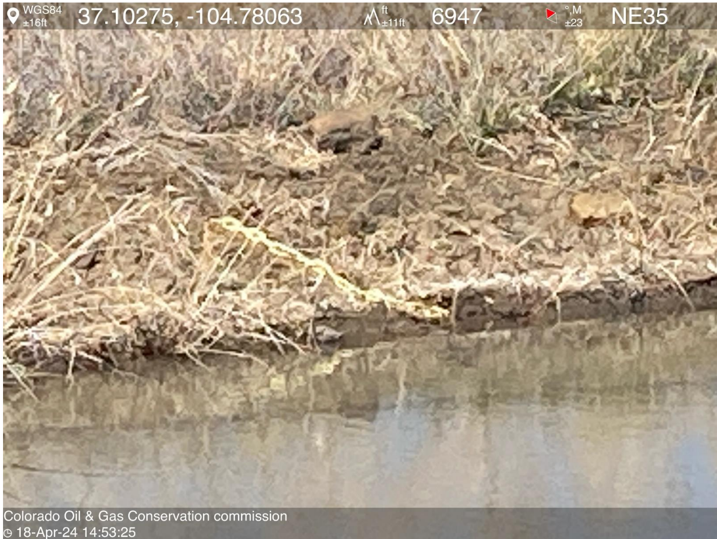
PHOTO 5: THE SALT/MINERAL DEPOSIT RING AROUND THE PIT INDICATES THAT THE PIT IS BEEING MAINTAINED ABOVE 2' FREEBOARD ON A REGULAR BASES, THE RULE STATES THAT THERE MUST BE A MINIMUM OF 2' FREEBOARD AT ALL TIMES. THIS MEANS THAT THE PIT MUST BE PULLED/DRAINED BEFORE FLUID LEVEL REACHES THE 2' FREEBOARD.
