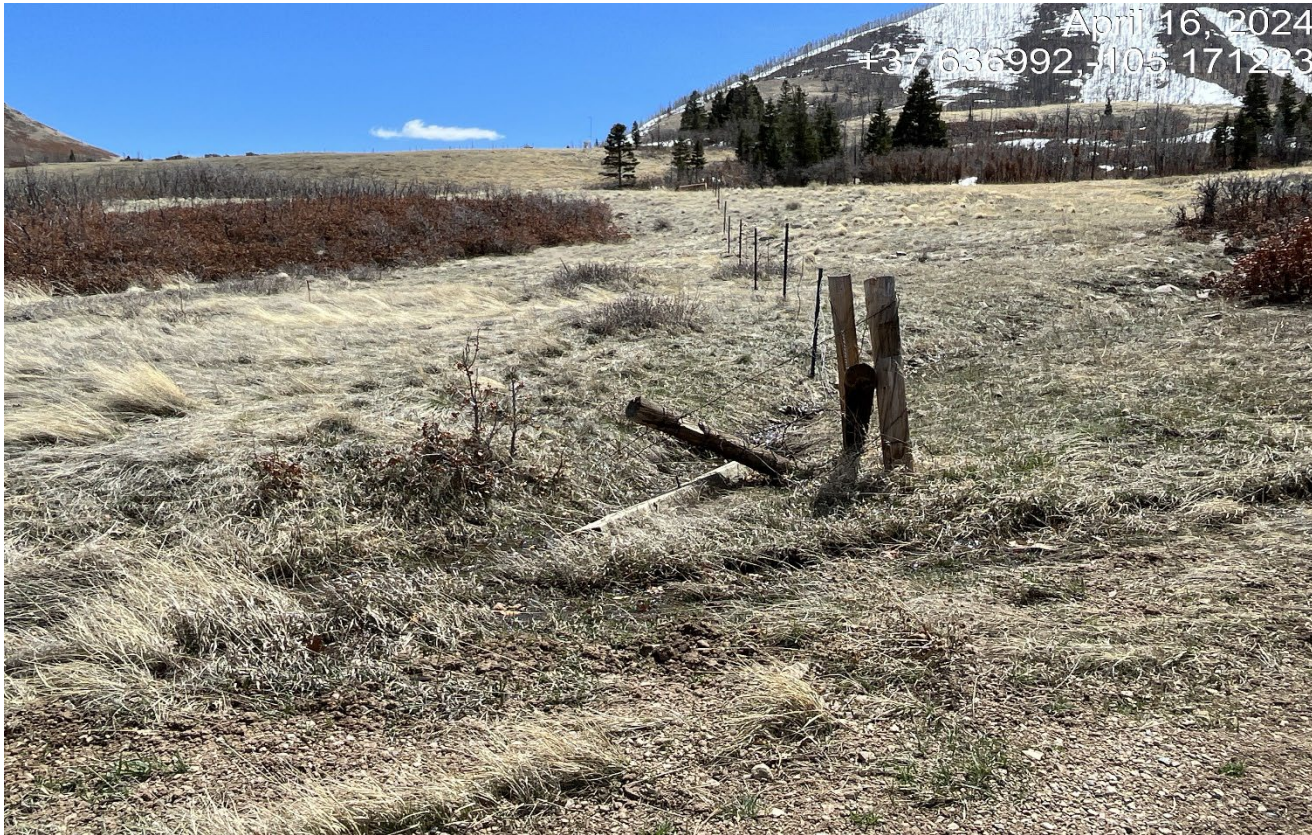
Photo 2. The perimeter fence around the location is not maintained and there are posts and wire laying on the ground.
