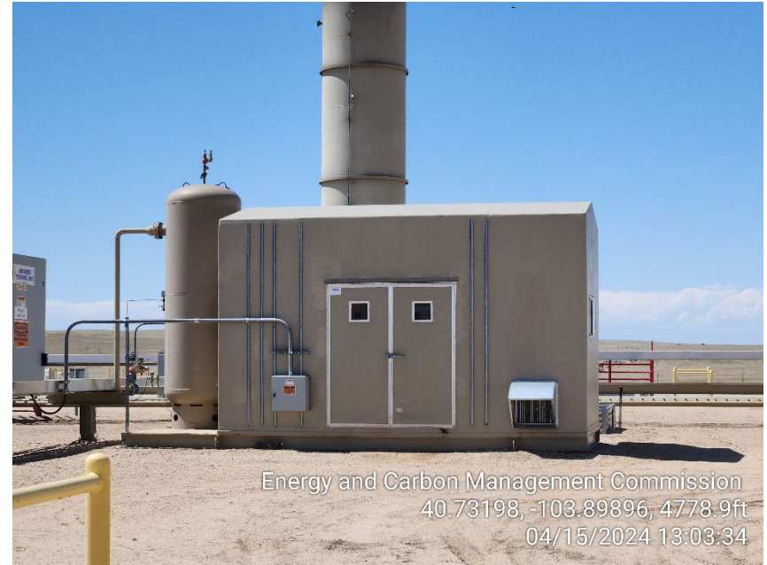
Photo 12 – Instrumental Air Unit
