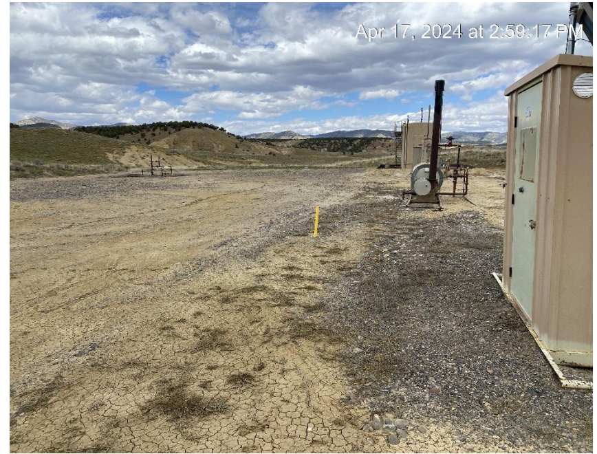
Location from Southwest corner
