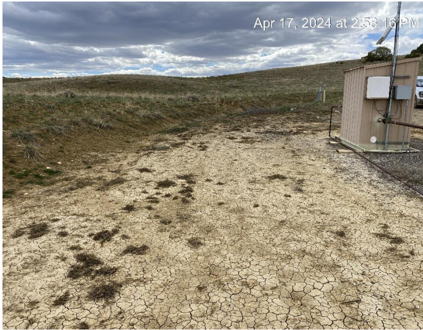
Sediment migration on location
