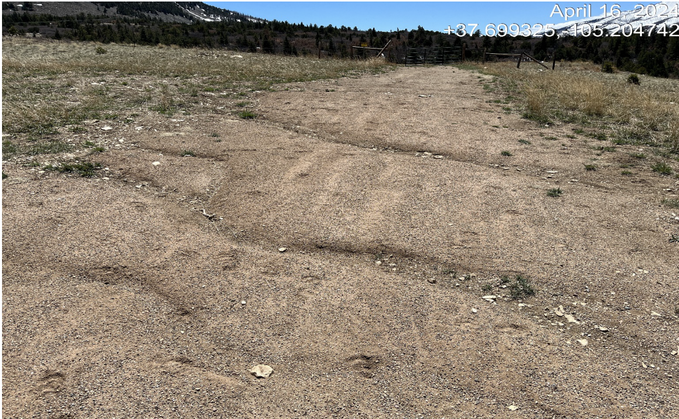
Photo 1. Facing south toward the access road. There is erosion occurring across the road and no BMP's were installed. The access road will need to be decompacted and reclaimed. Previous corrective action has not been completed.
