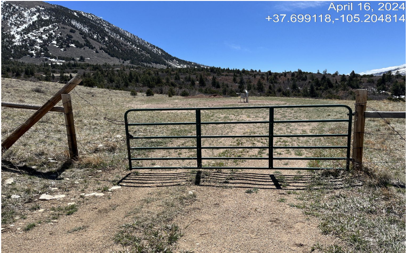
Photo 2. Facing south toward the location. The well has been plugged and abandoned . The location will need to be recontoured back to the original contours and reclaimed. This gate does not prevent livestock entry.
