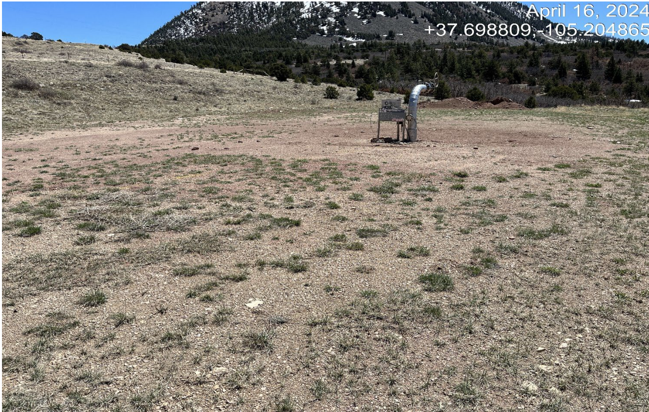
Photo 3. Facing toward the wellsite. The wellhead has been covered up and backfilled. This pipe riser must be removed. All equipment must be removed with 3 months of abandonment.
