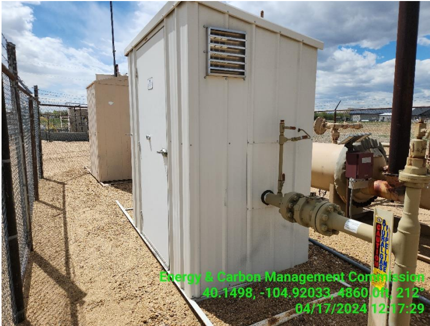
Photo 7 Gas Meter Run.
