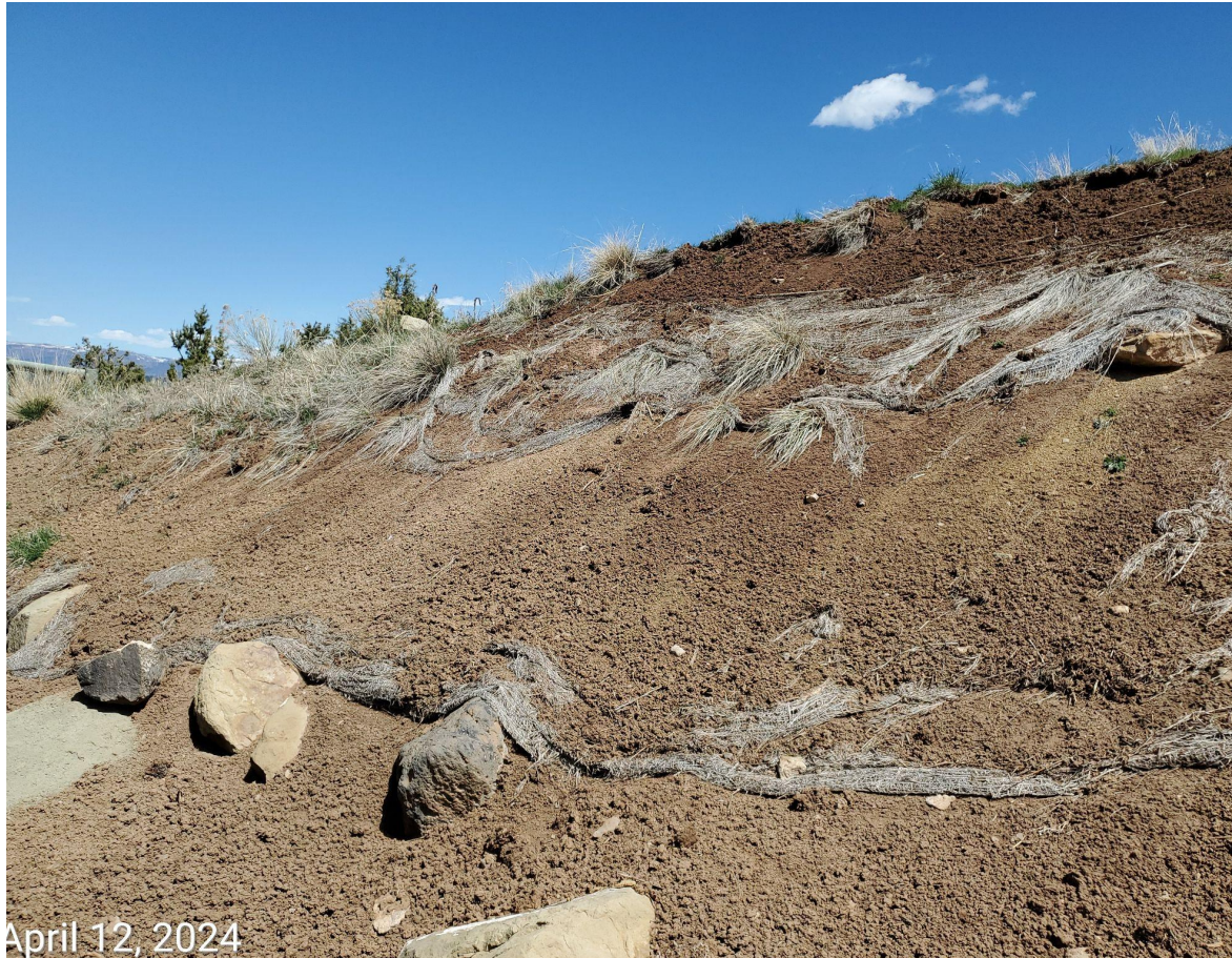
Photo 8: Continued from photo 7. Erosion blankets no longer in proper functioning condition. Stormwater and erosion control BMPs missing or insufficient.
