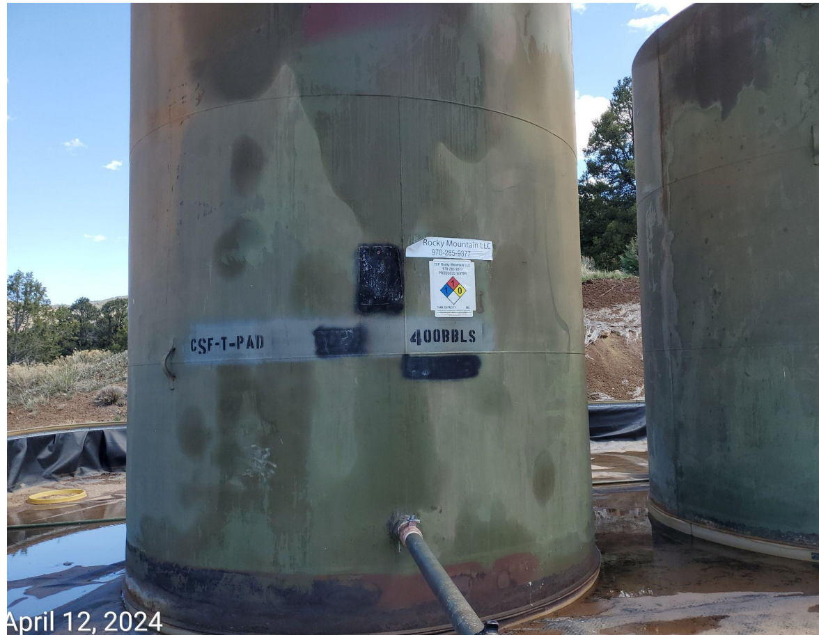
Photo 5: Tank label peeling. Maintenance advised.
