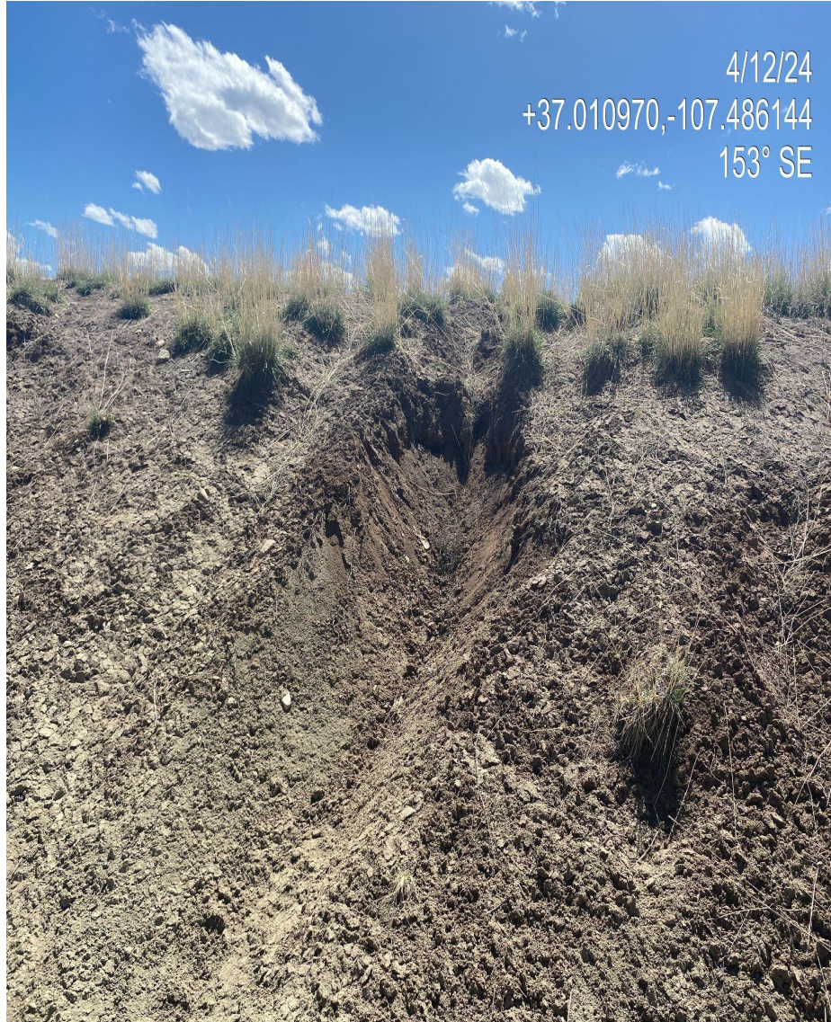
Photo 5. Gully erosion observed forming in the southern cut slope where soils remain unstabilized.
