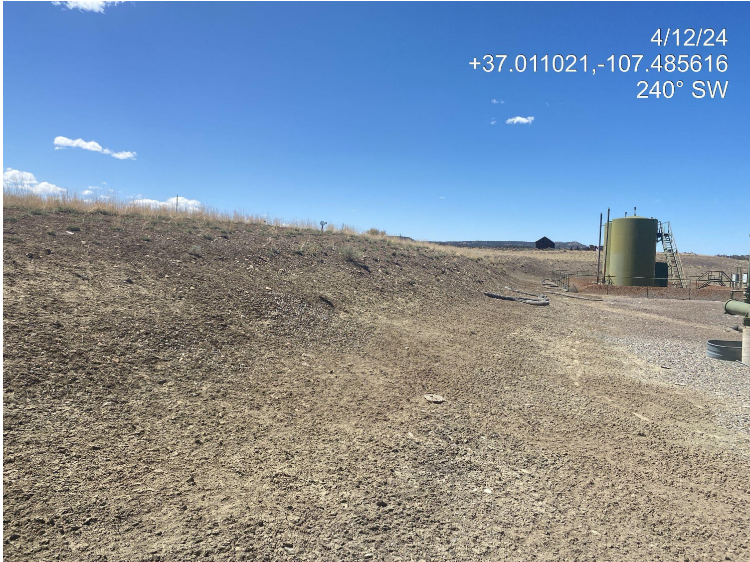
Photo 3. View of un stabilized southern cut slope/interim reclamation area. Erosion controls need to be installed until area is stabilized with perennial vegetation.
