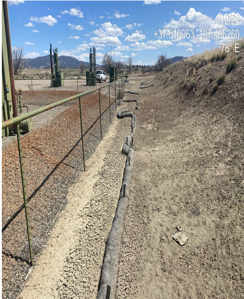
Photo 4. View of various piles of wattles in the southern portion of the disturbance that are no longer functioning and are considered debris.
