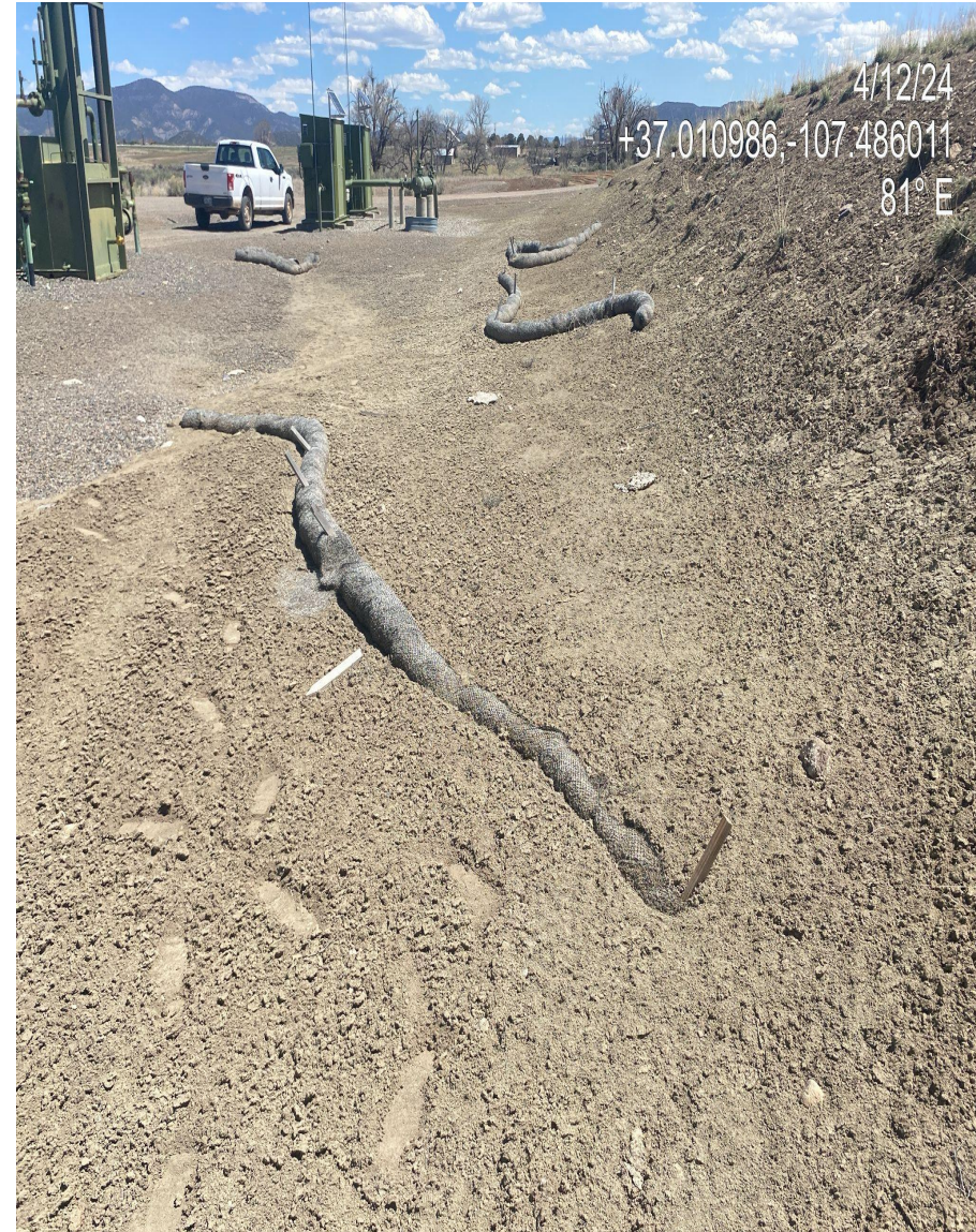
Photo 4. View of various piles of wattles in the southern portion of the disturbance that are no longer functioning and are considered debris.
