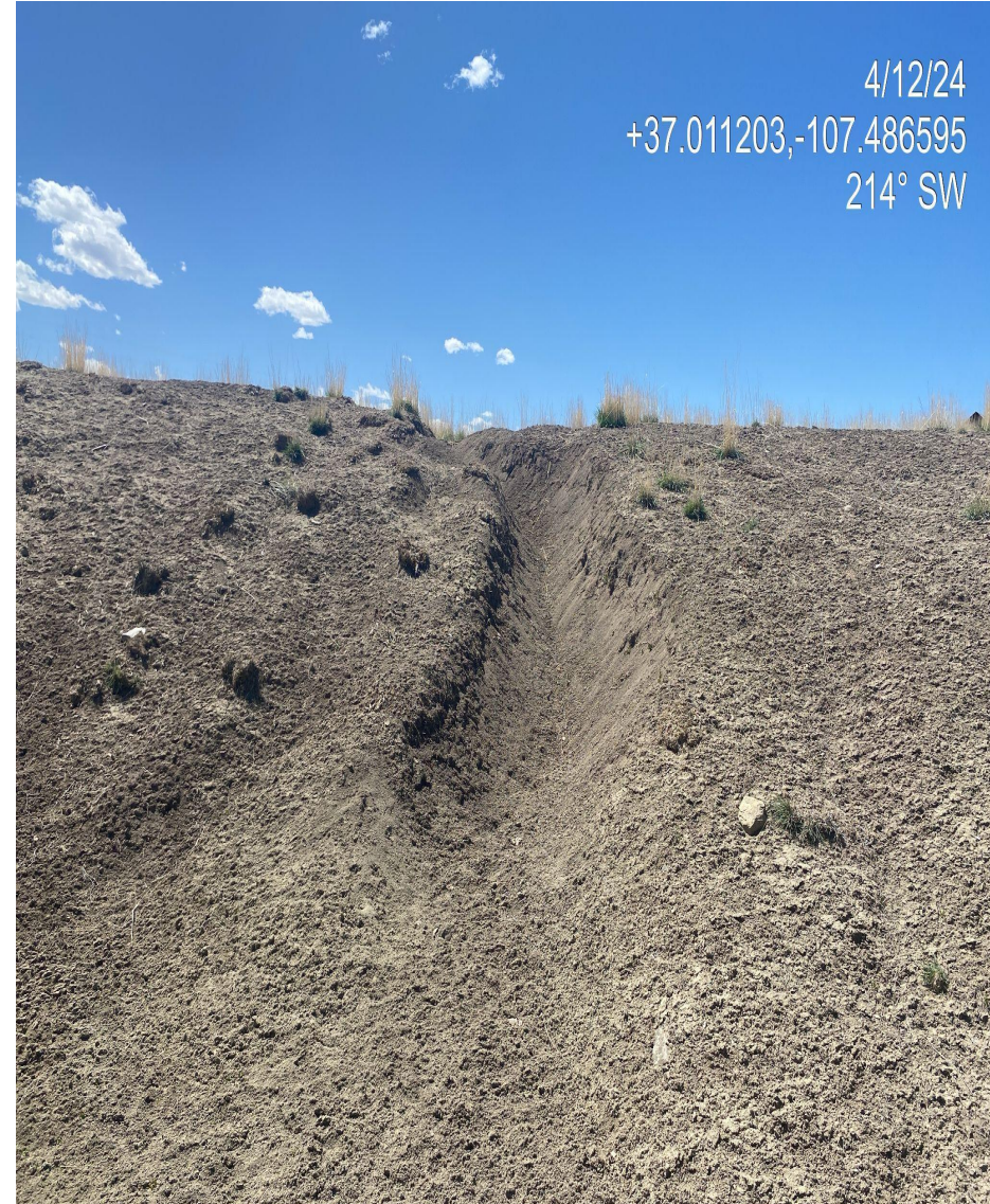
Photo 5. Gully erosion observed forming in the southern cut slope where soils remain unstabilized.
