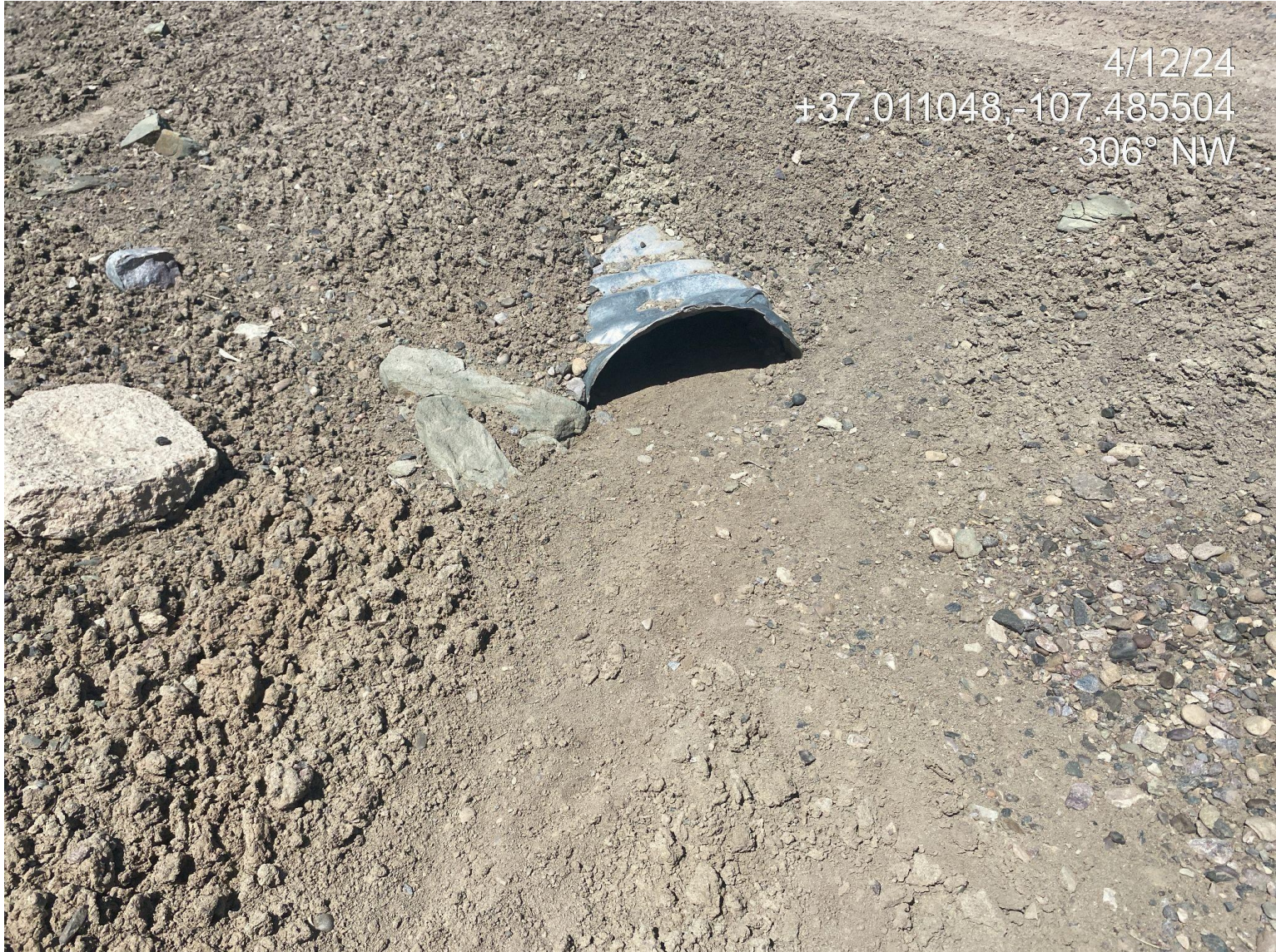
Photo 6. View of storm water culvert on location that is full of sediment and no longer functioning.
