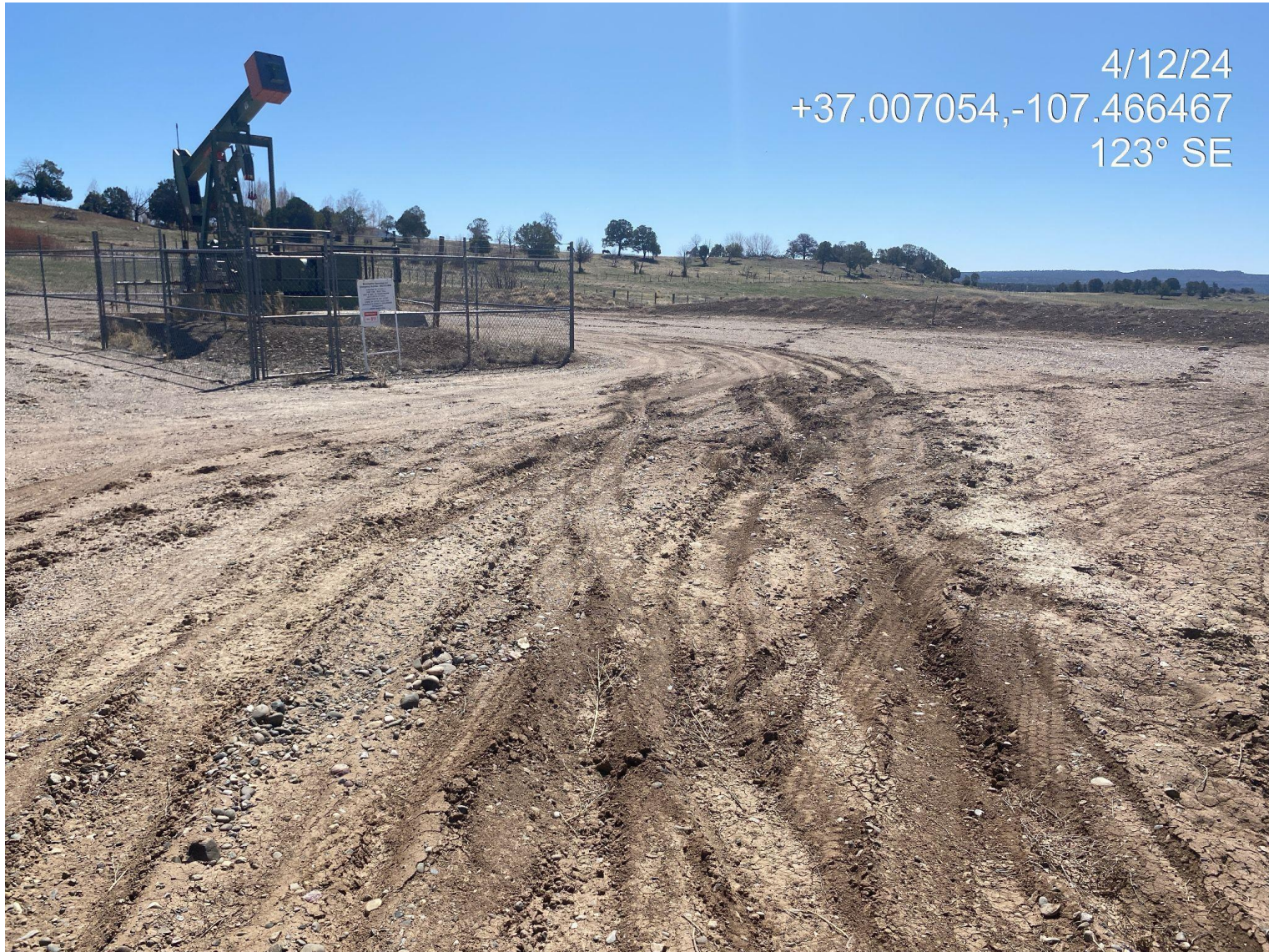
Photo 6. Rutting observed on location, additional stabilization is needed to minimize site degradation.
