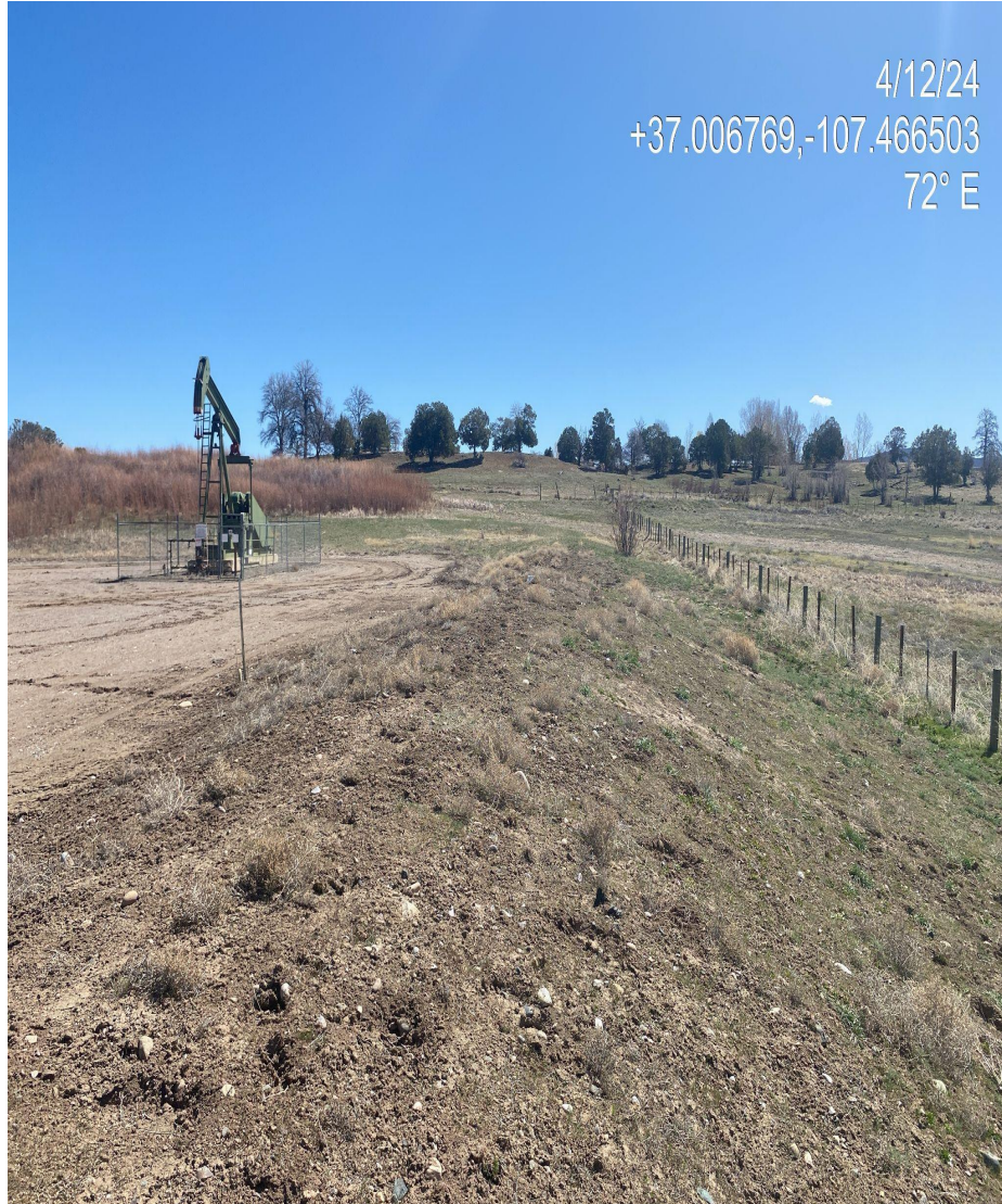
Photo 2. southern fill slope/interim reclamation areas dominated by kochia/russian thistle debris and lacking vegetation. Stormwater BMPs/soil stabilization is needed until long term stabilization is achieved with perennial vegetation.
