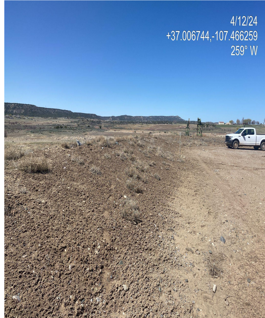
Photo 2. southern fill slope/interim reclamation areas dominated by kochia/russian thistle debris and lacking vegetation. Stormwater BMPs/soil stabilization is needed until long term stabilization is achieved with perennial vegetation.
