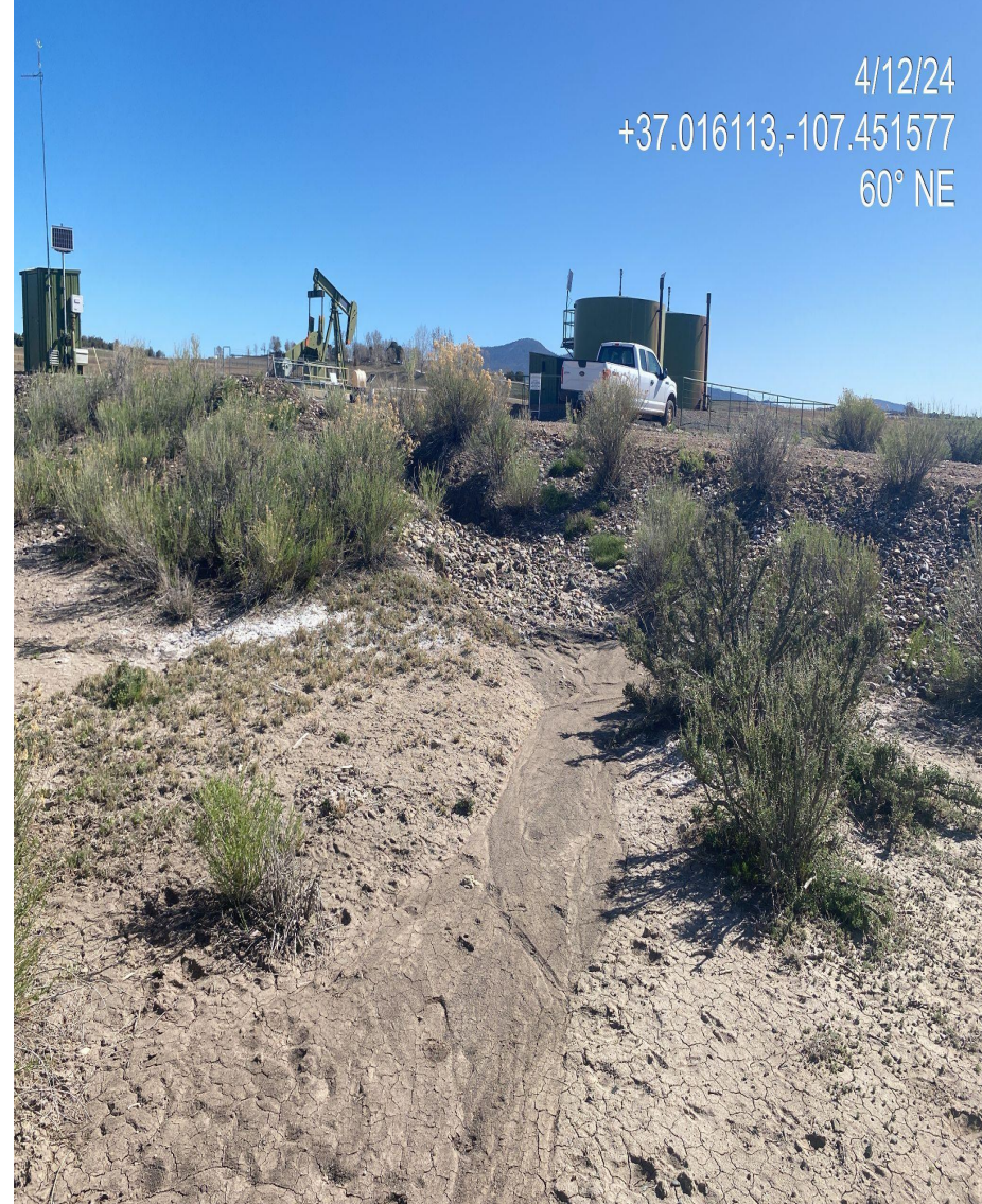
Photo 3. Evidence of sediment transport moving off location. Current storm water BMPs installed along the western edge of the access road at the access point are inadequate and not functioning properly.
