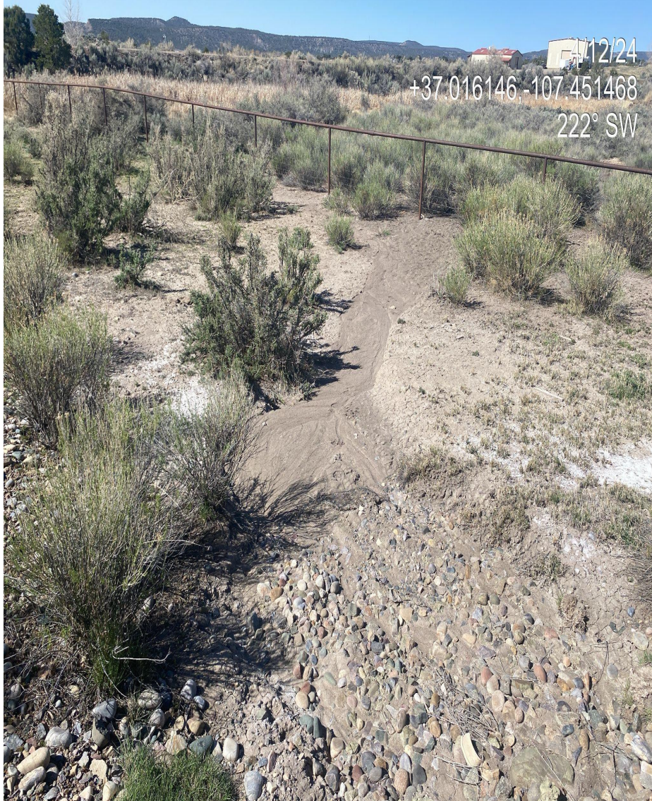
Photo 3. Evidence of sediment transport moving off location. Current storm water BMPs installed along the western edge of the access road at the access point are inadequate and not functioning properly.
