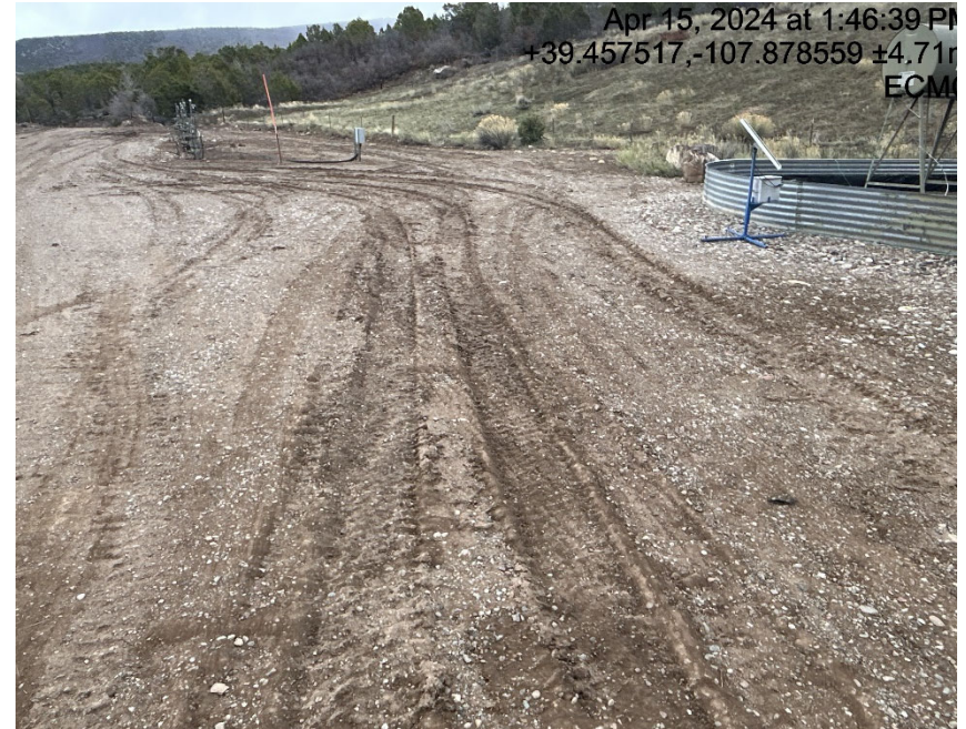
Some areas of lack of stabilization/compaction
