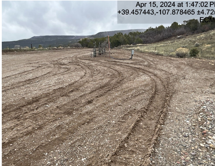
Some areas of lack of stabilization/compaction
