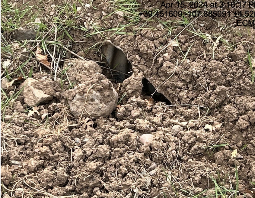
Culvert needs maintained
