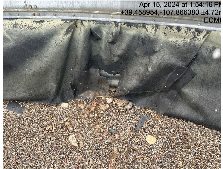
Holes in containment
