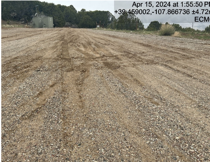
Some areas of lack of compaction/stabilization
