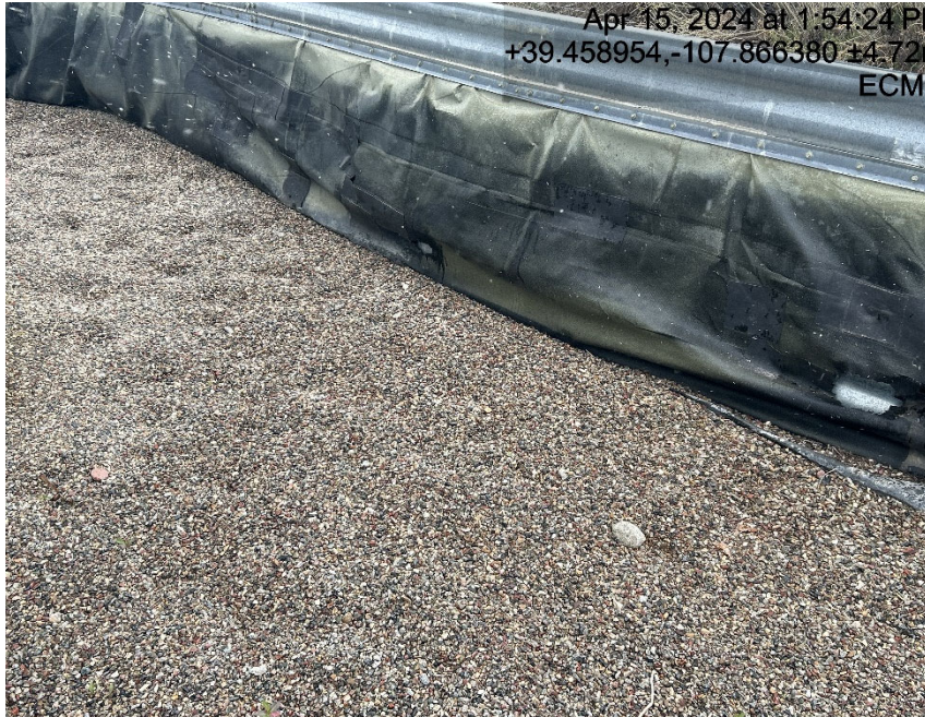
Holes in containment
