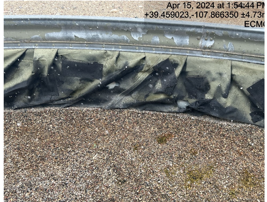
Holes in containment
