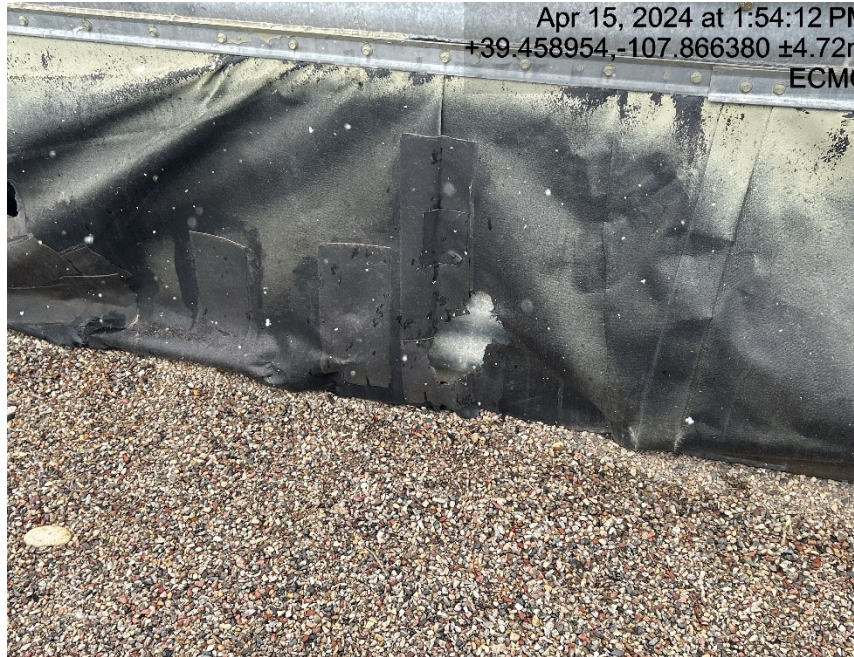
Holes in containment
