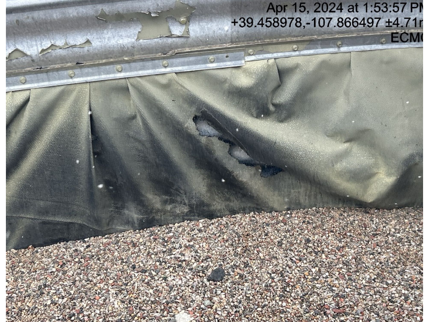
Holes in containment
