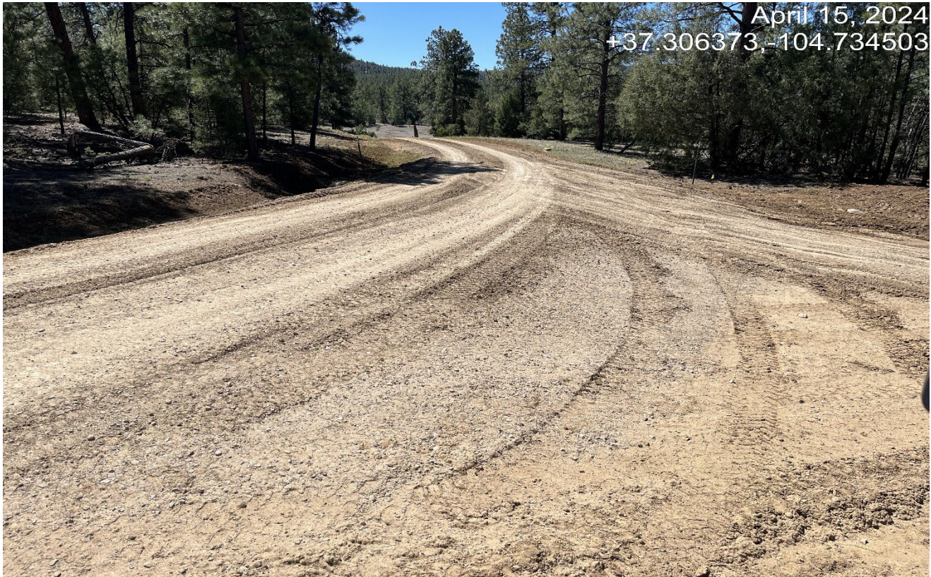
Photo 1. Facing south along the access road. A culvert was installed at this intersection for proper drainage.
