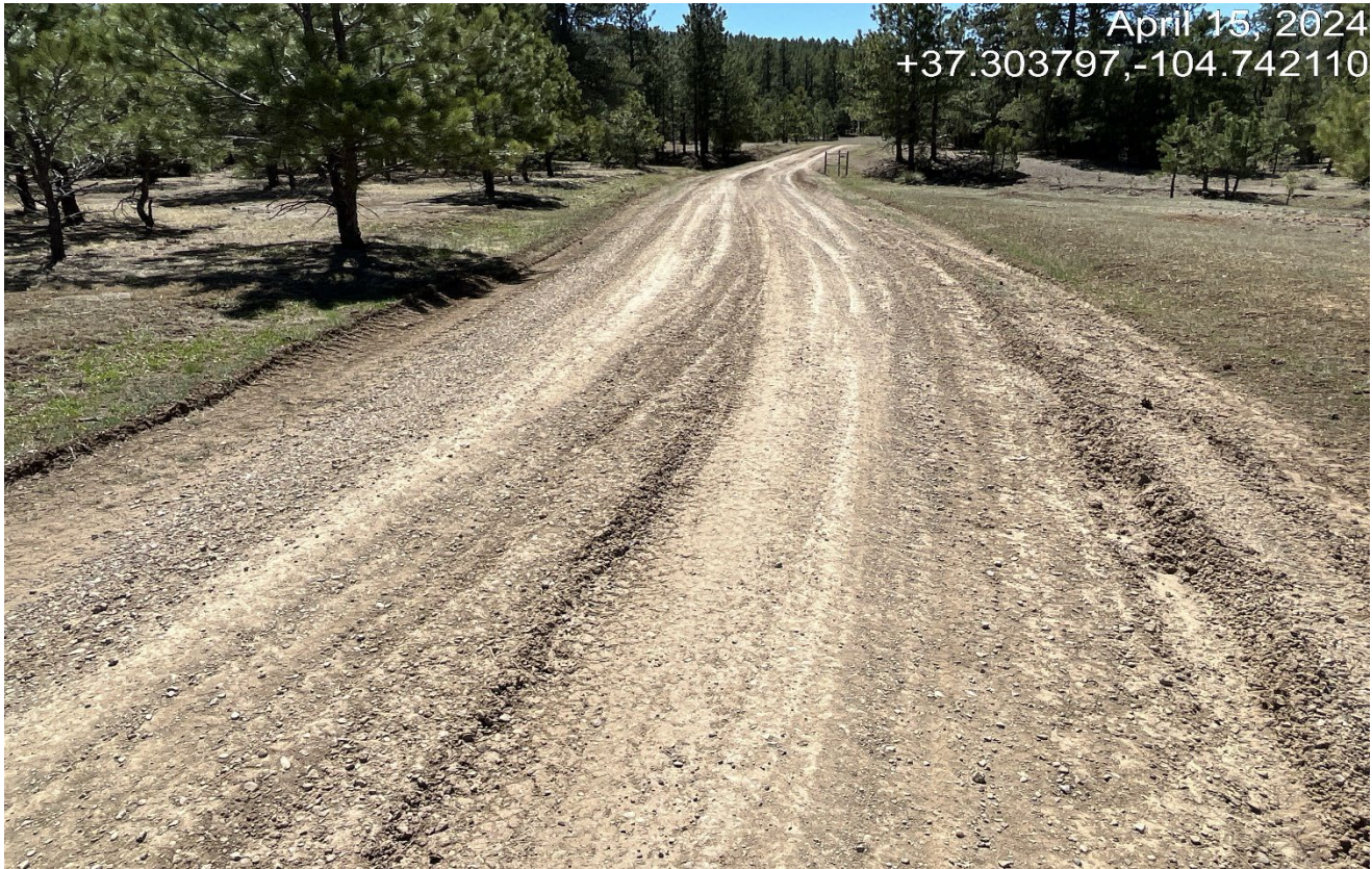
Photo 2. The access road has been repaired with additional gravel.
