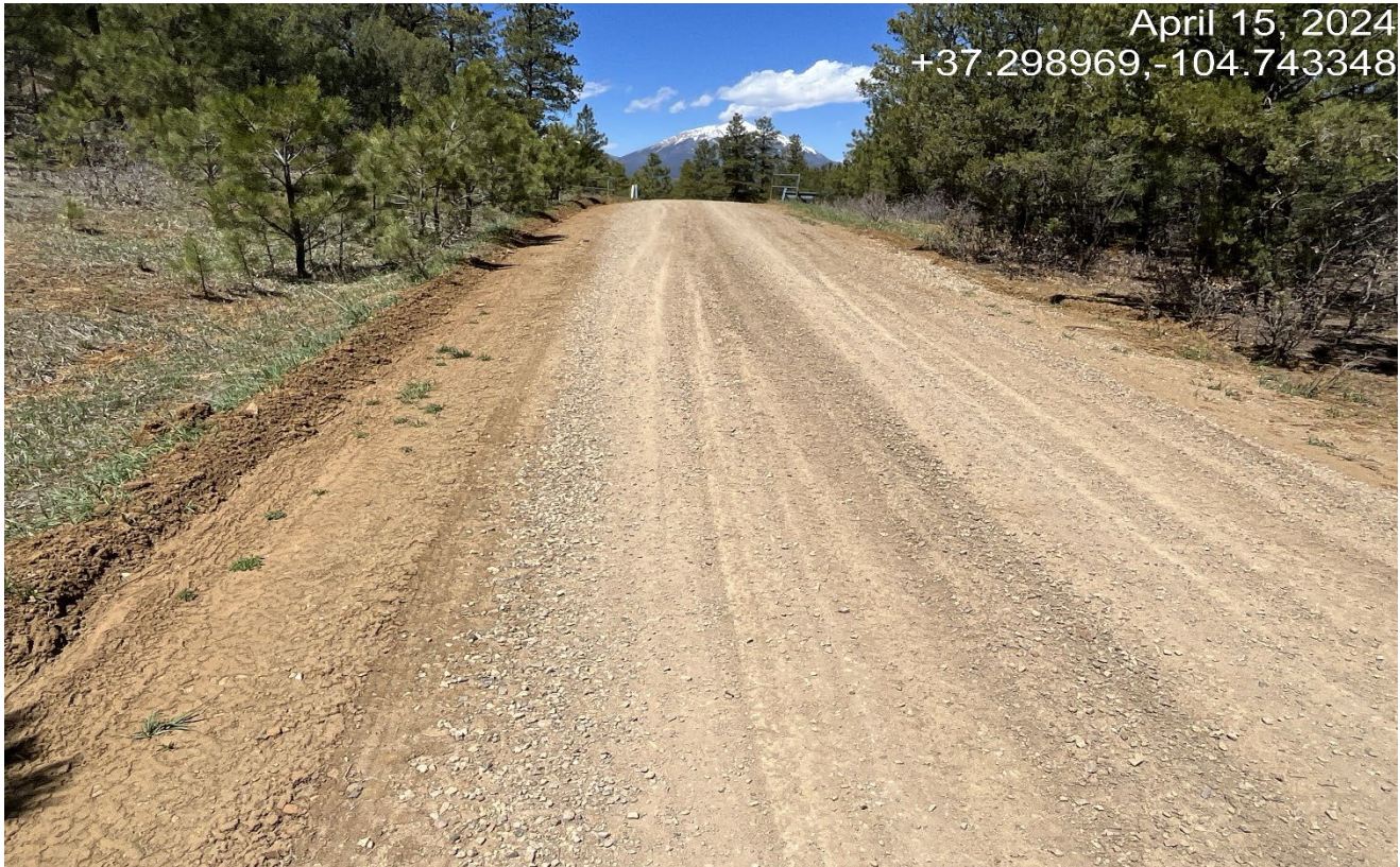
Photo 1. Facing northwest along the access road. The access road has been stabilized with additional road base.
