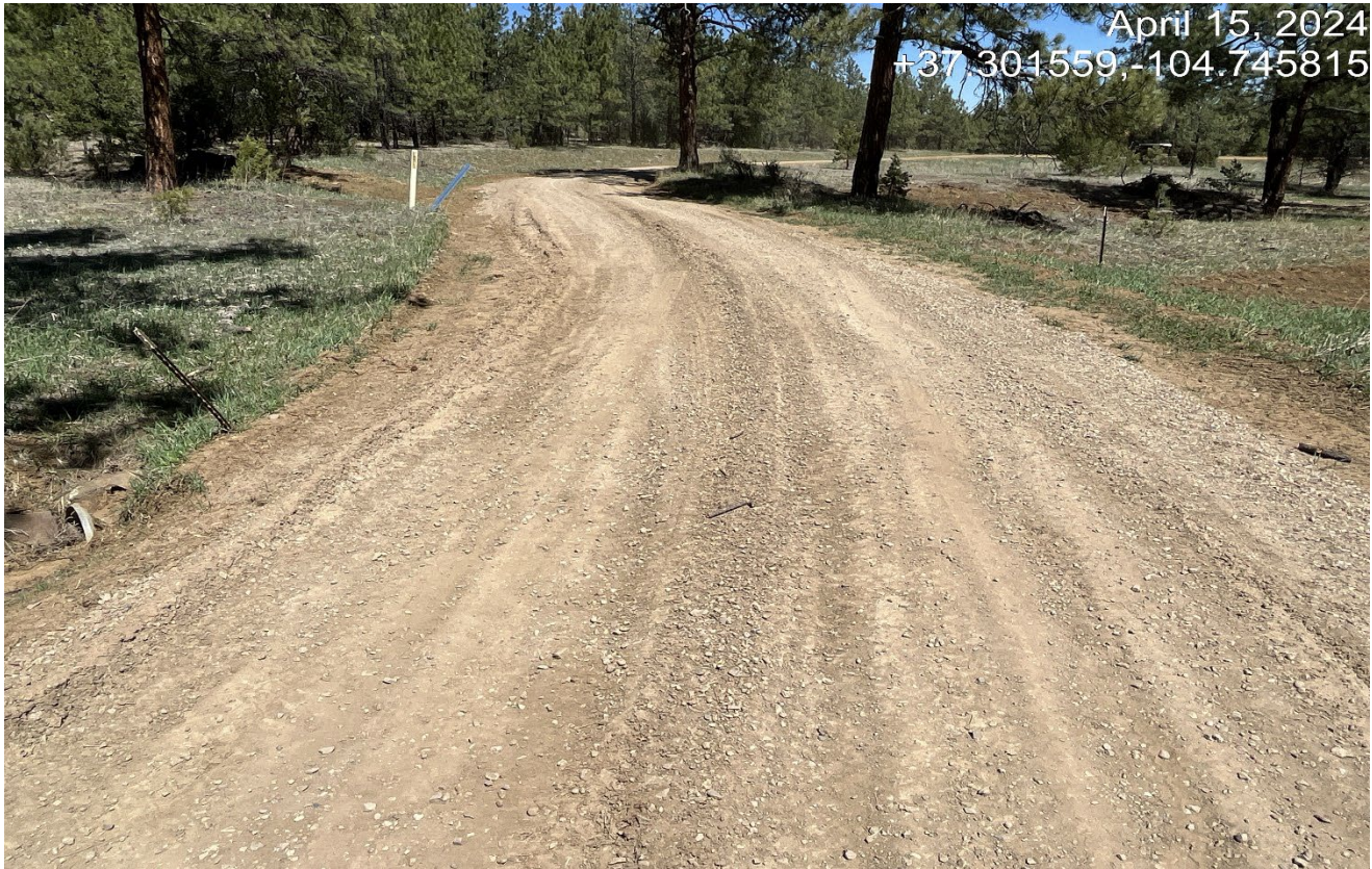
Photo 3. The access road has been repaired with additional gravel.
