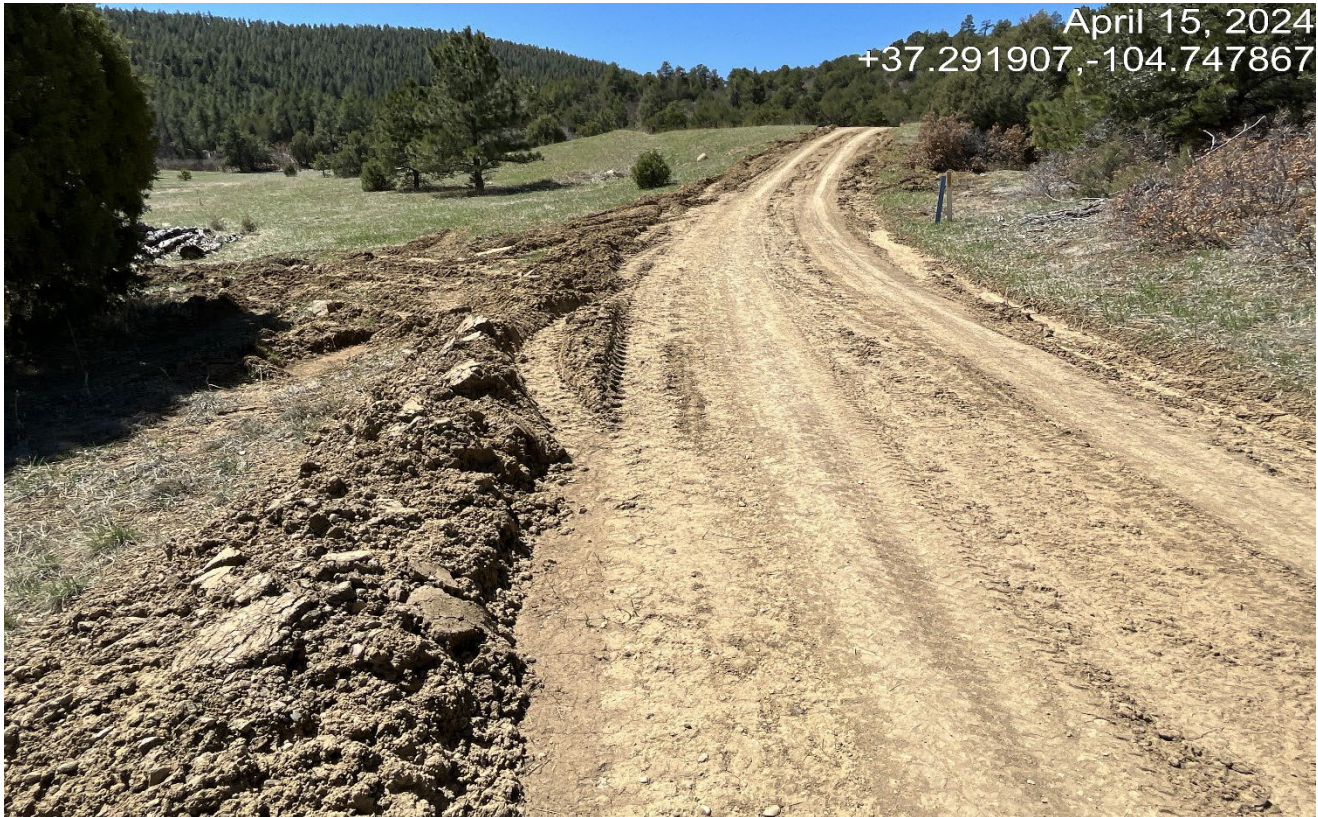
Photo 1. Facing southwest along access road. The access road is not stabilized and it appears a vehicle went off the road causing rutting disturbance that will need to be repaired.
