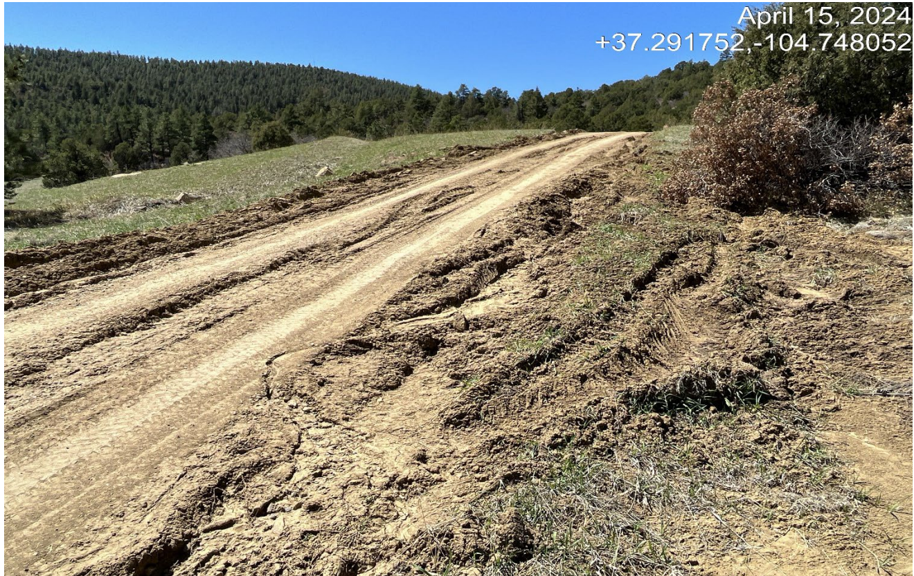
Photo 2. There is erosion and vehicle rutting near the location that needs to be repaired..
