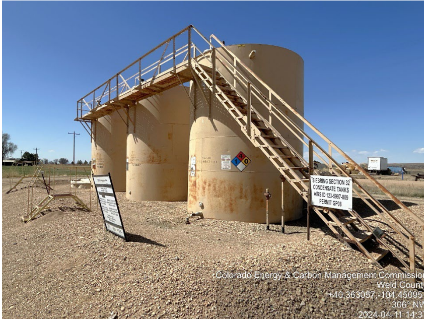
Photo #3 Siebring 41-32, 31-32, 32-32, 42-32, CNE-32 Battery site Inactive | Shut-down Tank(s): SE corner
