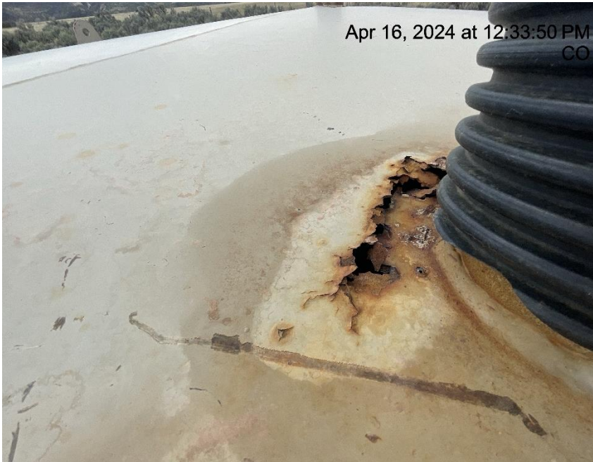
Photo # 4191 Possible tank failure – tank appears to be compromised, holes & corrosion on the top of tank
