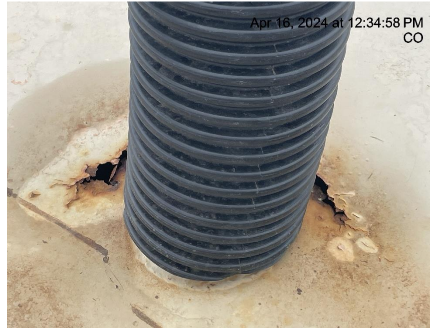
Photo # 4188 Possible tank failure – tank appears to be compromised, holes & corrosion on the top of production tank
