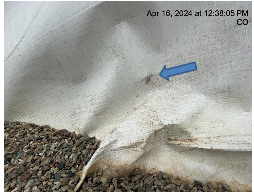
Photo # 4196 Hole in liner/liner needs maintenance
