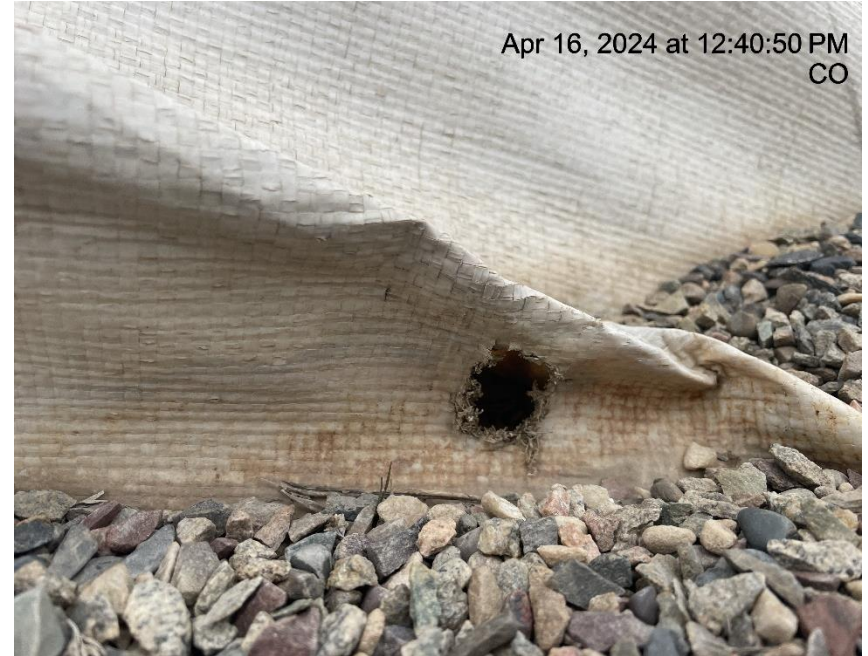
Photo # 4194 Hole in liner/liner needs maintenance
