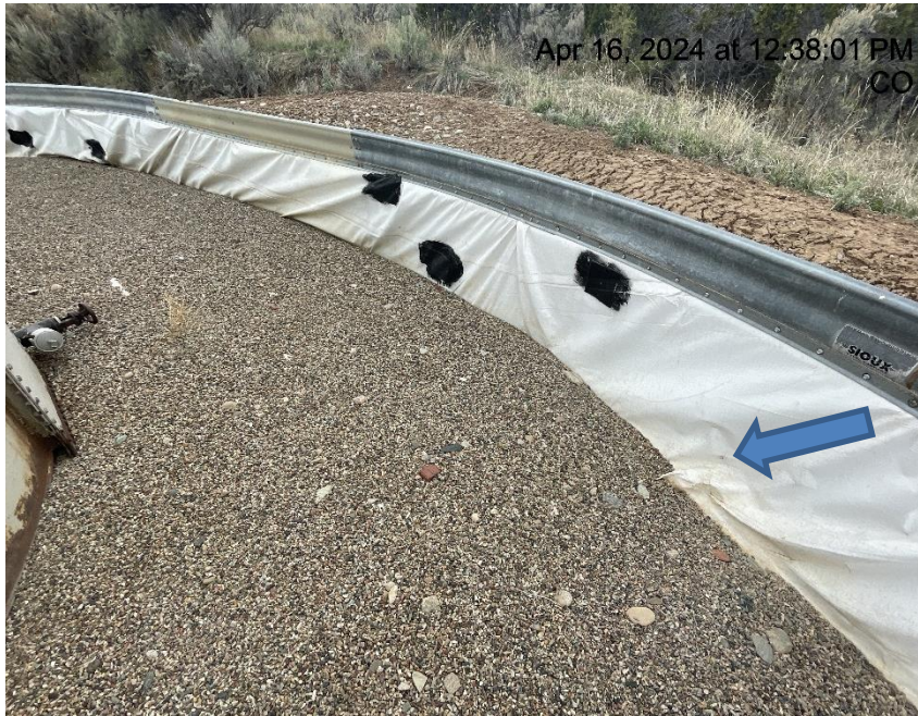
Photo # 4195 Hole in liner/liner needs maintenance
