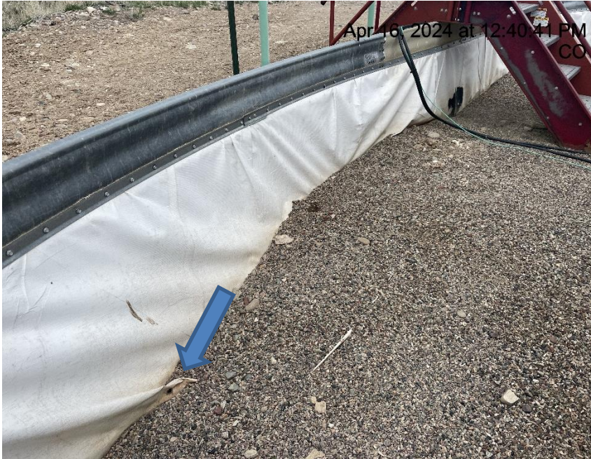
Photo # 4193 Hole in liner/liner needs maintenance
