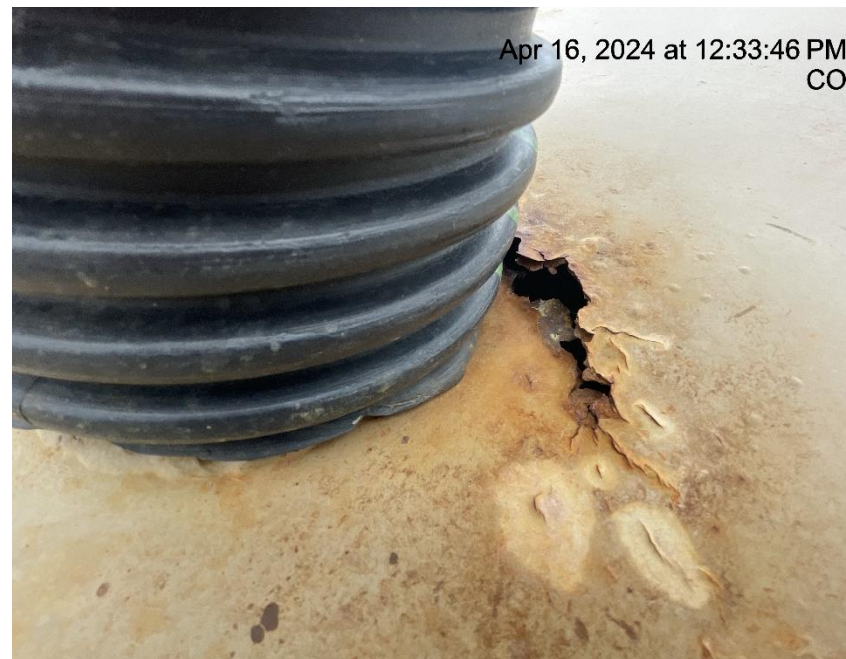
Photo # 4190 Possible tank failure – tank appears to be compromised, holes & corrosion on the top of tank
