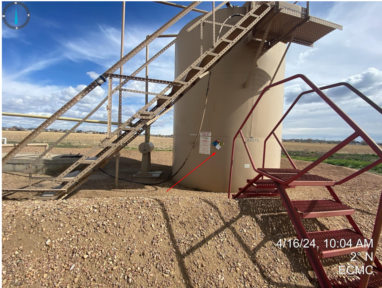
Photo 2. NFPA placard at tank is peeling/faded/cracked.
