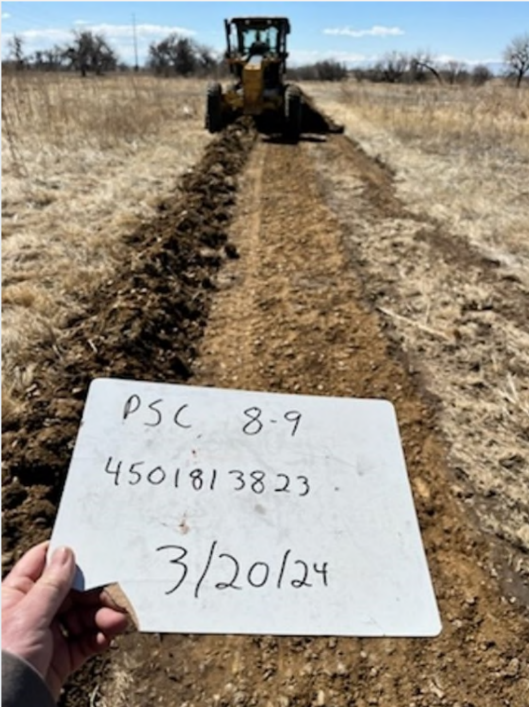
Photo Name: Remove roadbase
