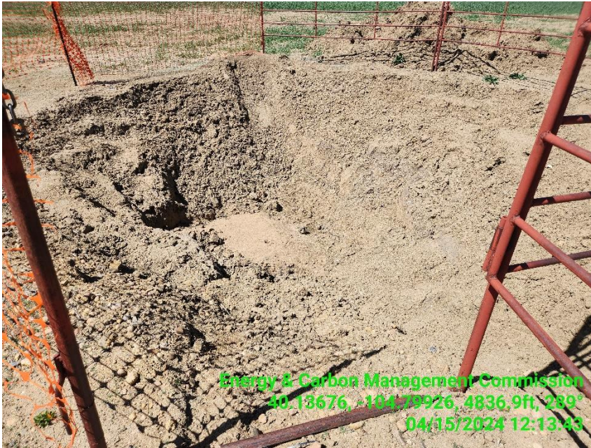
Photo 3 PA excavation, cut & cap.
