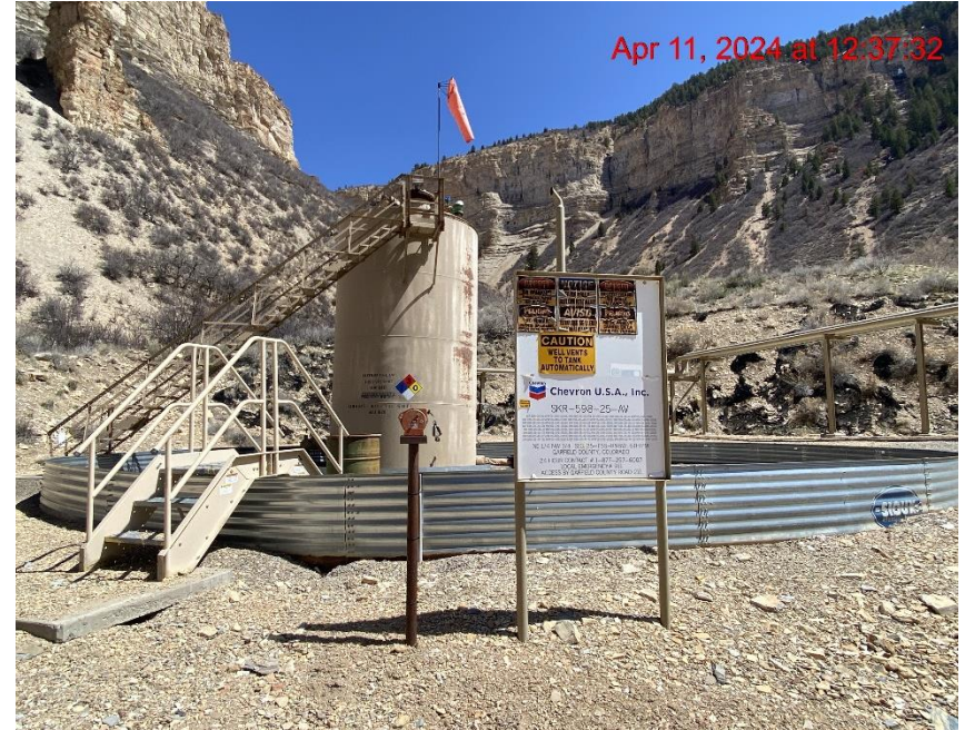
Tank Battery – Photo #00583
