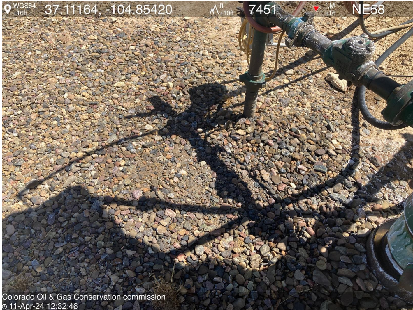
PHOTO 4: AREA OF IMPACTED SOIL NEAR DRIVEHEAD (HYDRAULIC OIL IS LEAKING FROM DRIVE MOTOR). Conduct maintenance on equipment, cleanup stained material and review self inspection processes. COMPLY WITH RULE 1002,.(2).D. CA DATE 4-18-2024.
