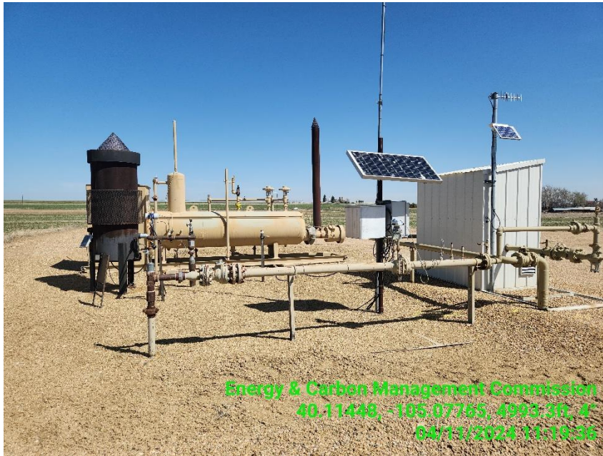
Photo 5 Gas Meter Run, card indicates current calibration. ECD & Horizontal Heated Separator.
