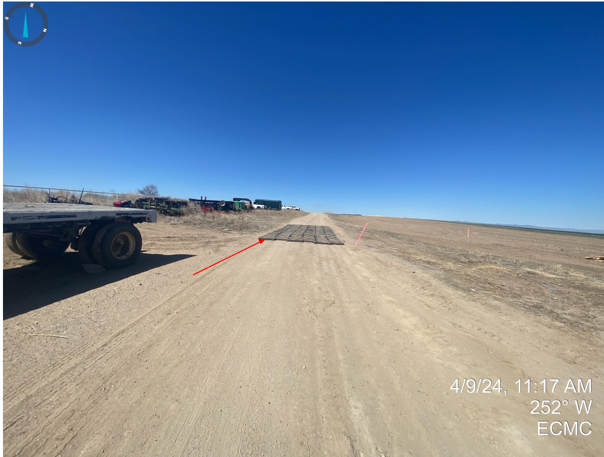
Photo 2. Vehicle track out pad installed along the access road.
