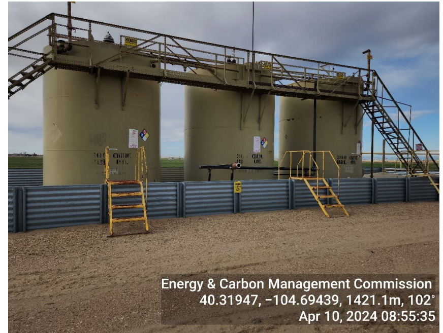
Photo 6: Tank Battery
