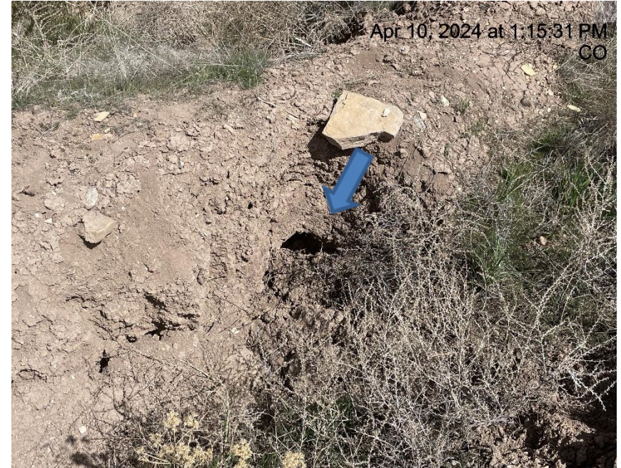
Photo # 3465 Tunnel erosion in ditch/BMP needs maintenance (ditch is near sediment trap along lease road approximately 70 yards from entrance to location)
