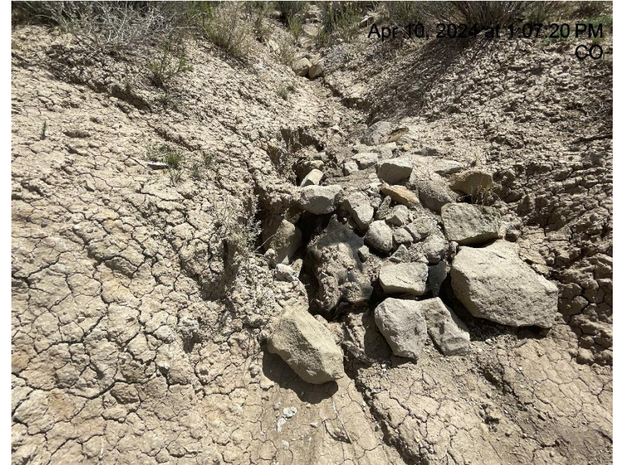
Photo # 3467 Rip Rap/BMP on sediment trap inlet needs maintenance - stormwater is cutting/eroding around edge of Rip Rap. (N/NW area of location)
