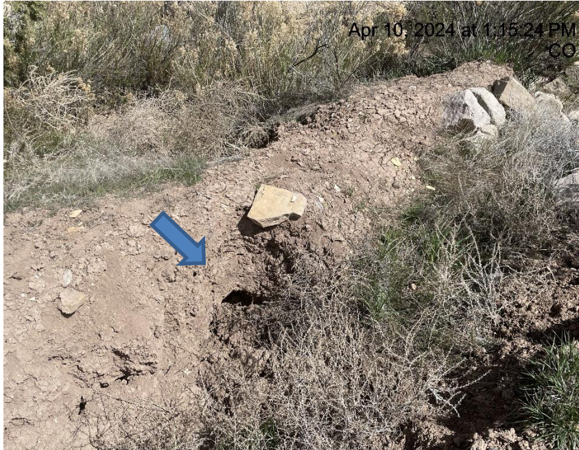
Photo # 3464 Tunnel erosion in ditch/BMP needs maintenance (ditch is near sediment trap along lease road approximately 70 yards from entrance to location)
