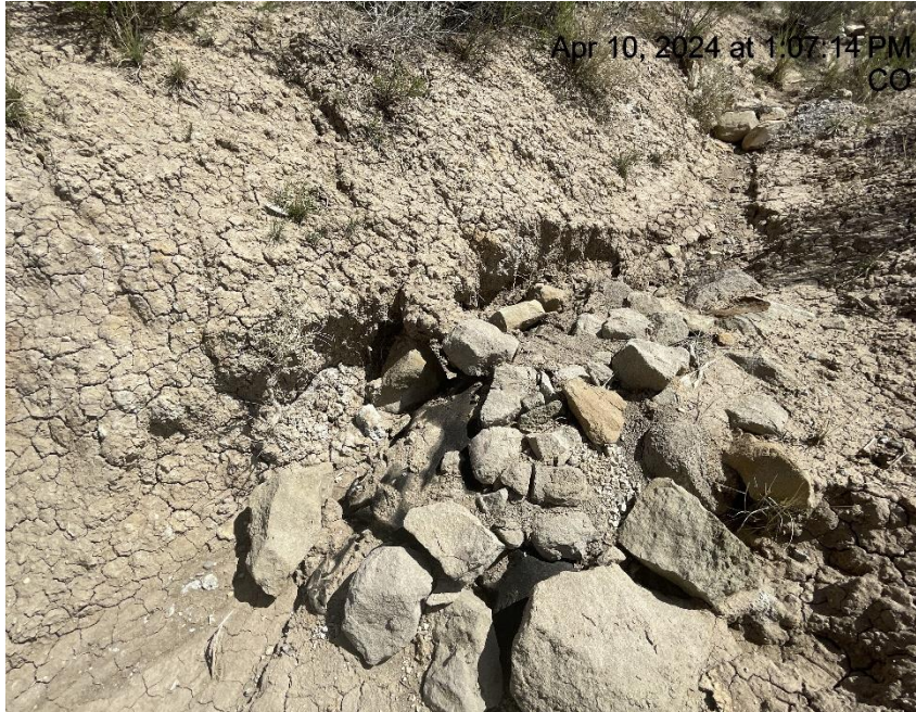
Photo # 3466 Rip Rap/BMP on sediment trap inlet needs maintenance - stormwater is cutting/eroding around edge of Rip Rap. (N/NW area of location)
