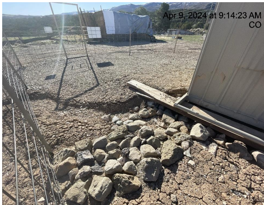
Photo # 3184 Rip Rap Run/BMP needs maintenance
