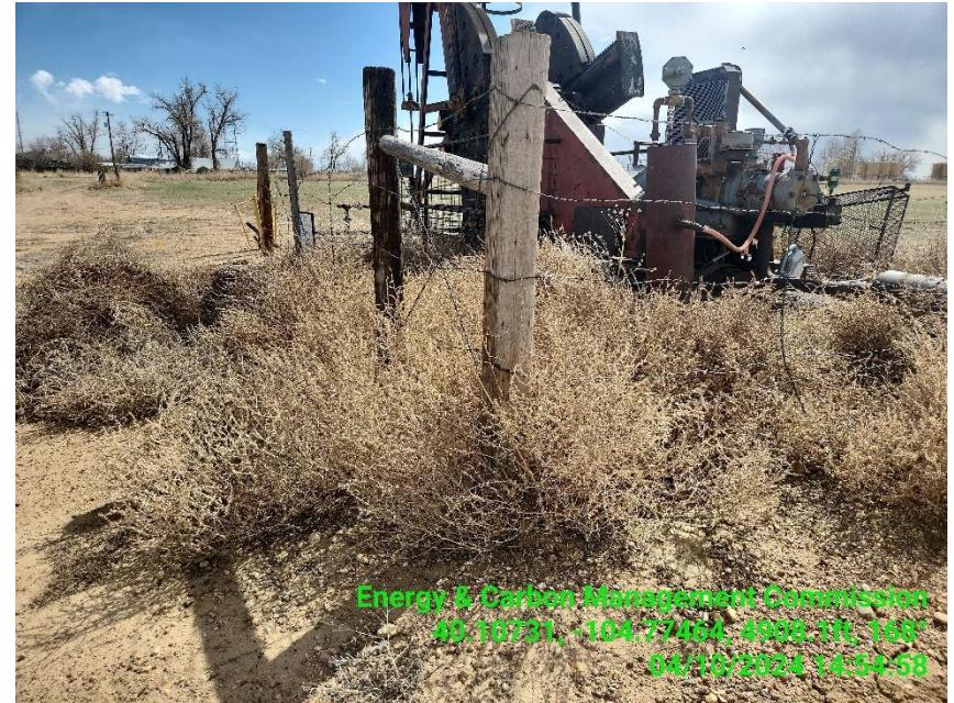
Photo 12 Pump jack base is over run with debris (dead vegetation)..
