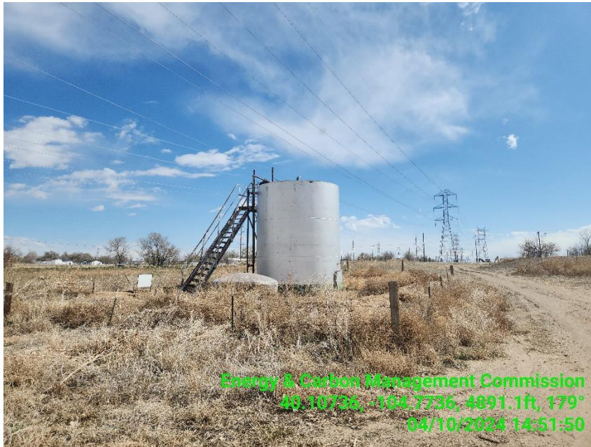
Photo 3 TB berm is over run with debris (dead vegetation).
