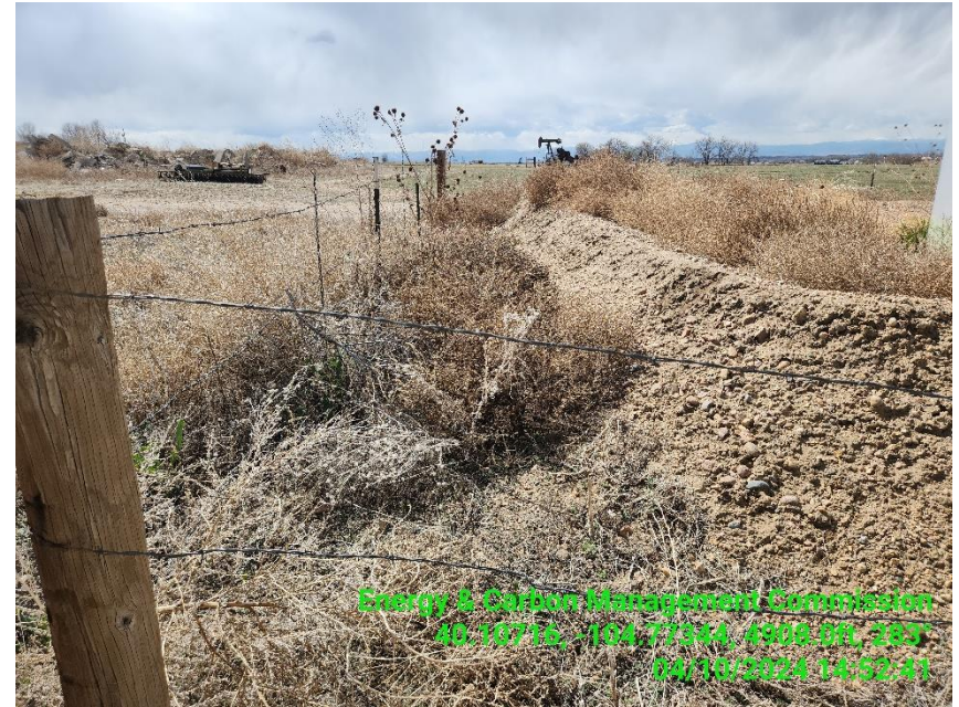
Photo 6 TB berm over run with debris (dead vegetation).
