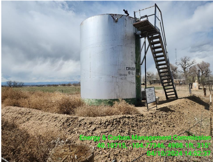
Photo 5 TB berm over run with debris (dead vegetation).
