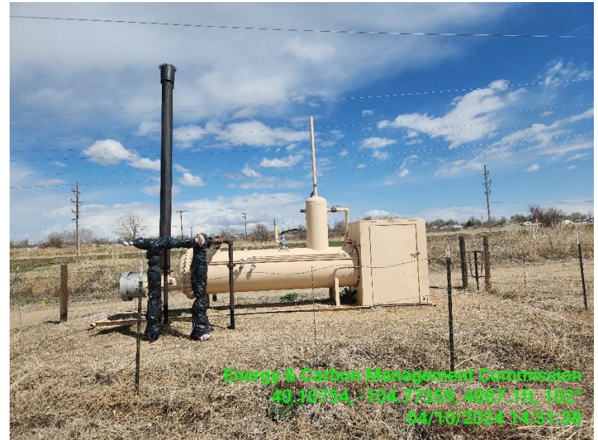
Photo 2 Horizontal heated Separator.
