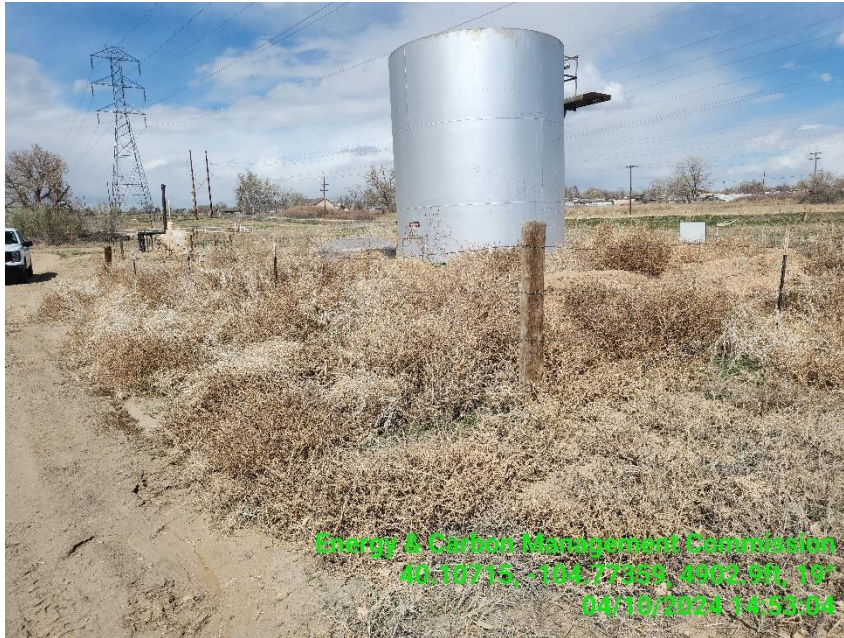
Photo 7 TB berm over run with debris (dead vegetation).
