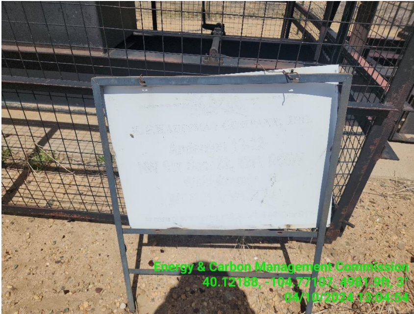
Photo 3 WH sign completely faded.
